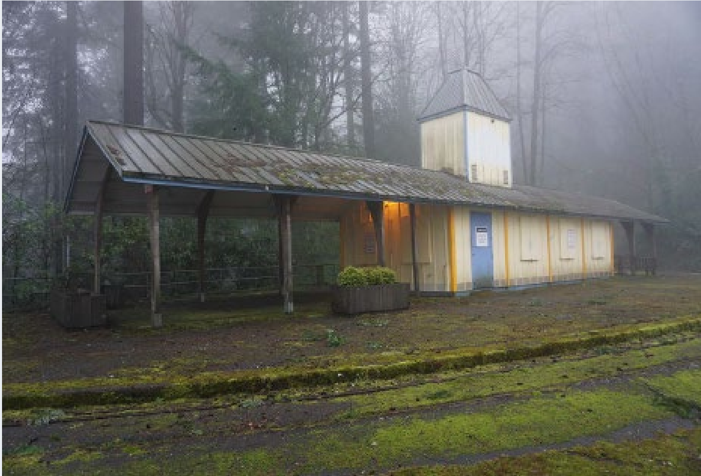
Washington Park Station looking Southwest Today
