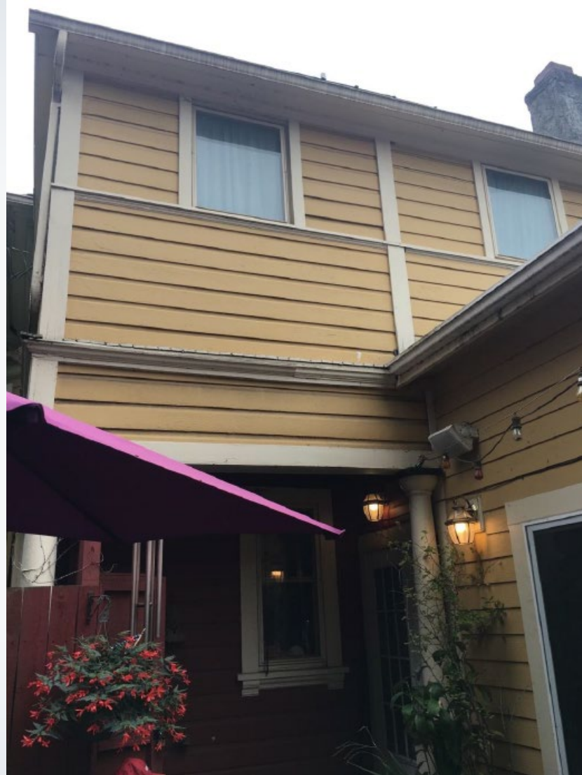
Enclosed Sleeping Porch and Kitchen Addition (right) Today
