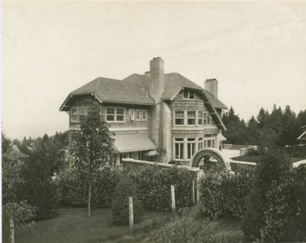
Keating Residence West Wall and South Façade (date unknown)
