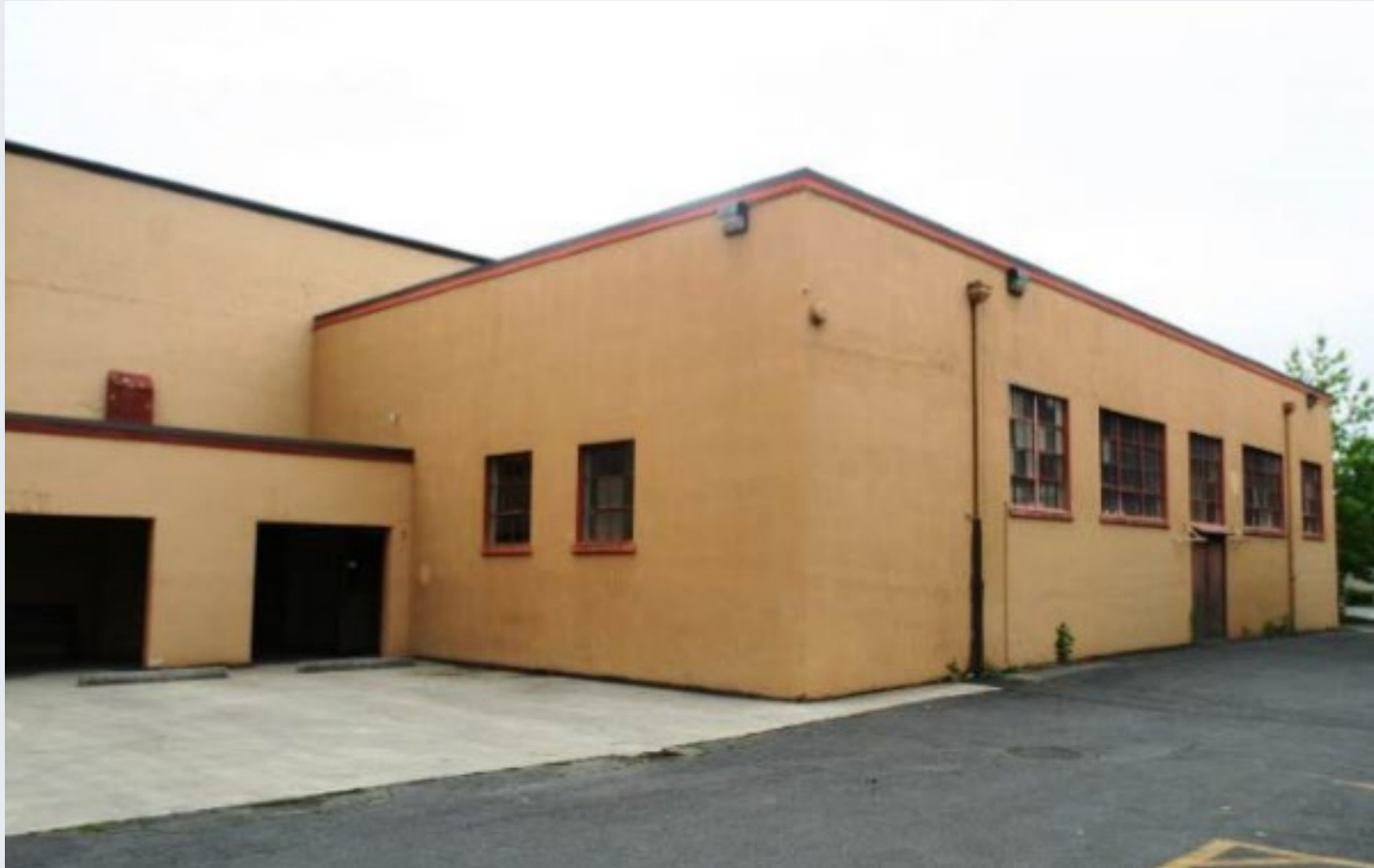
Multnomah School West Elevation of 1923 School (left) and 1925 Girl's Gymnasium (right) Today
