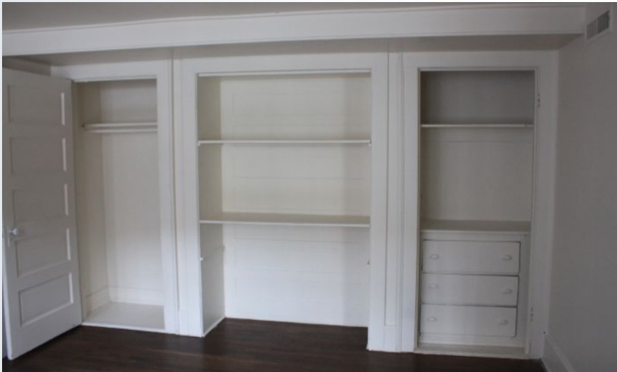
Wheeldon Annex Interior Details Today - Elevator and Built-in Furniture
