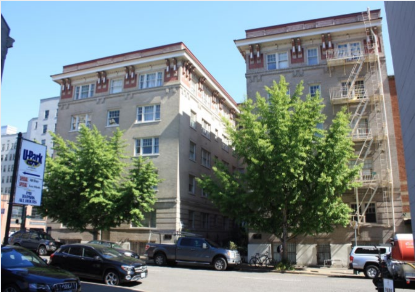
Wheeldon Annex South Elevation Today
