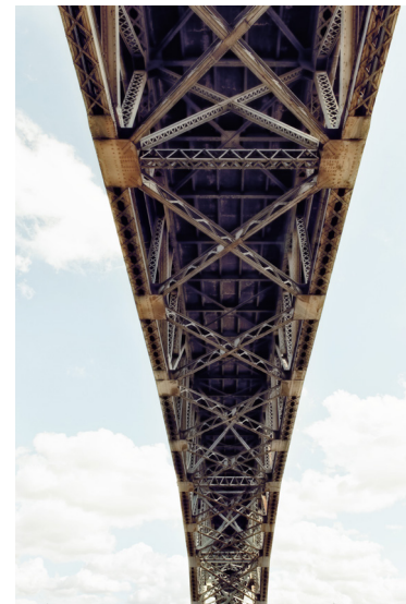
Ross Island Bridge
