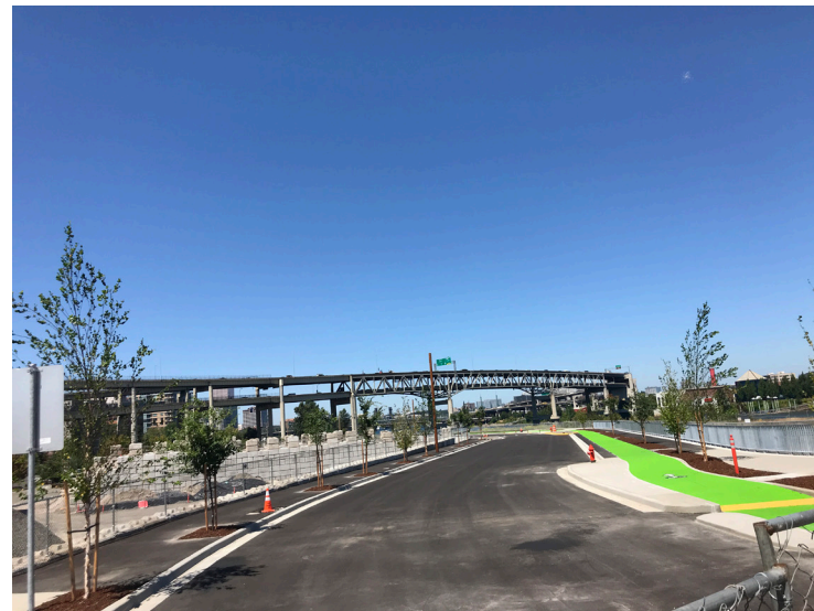
Future Bond Street recently completed
