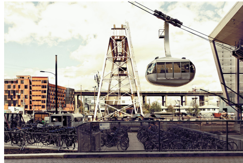
OHSU Aerial Tram with Zidell Crane in background
