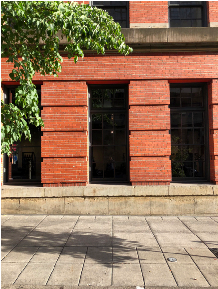
4. Crane Flats and Lofts Striated brick pattern
