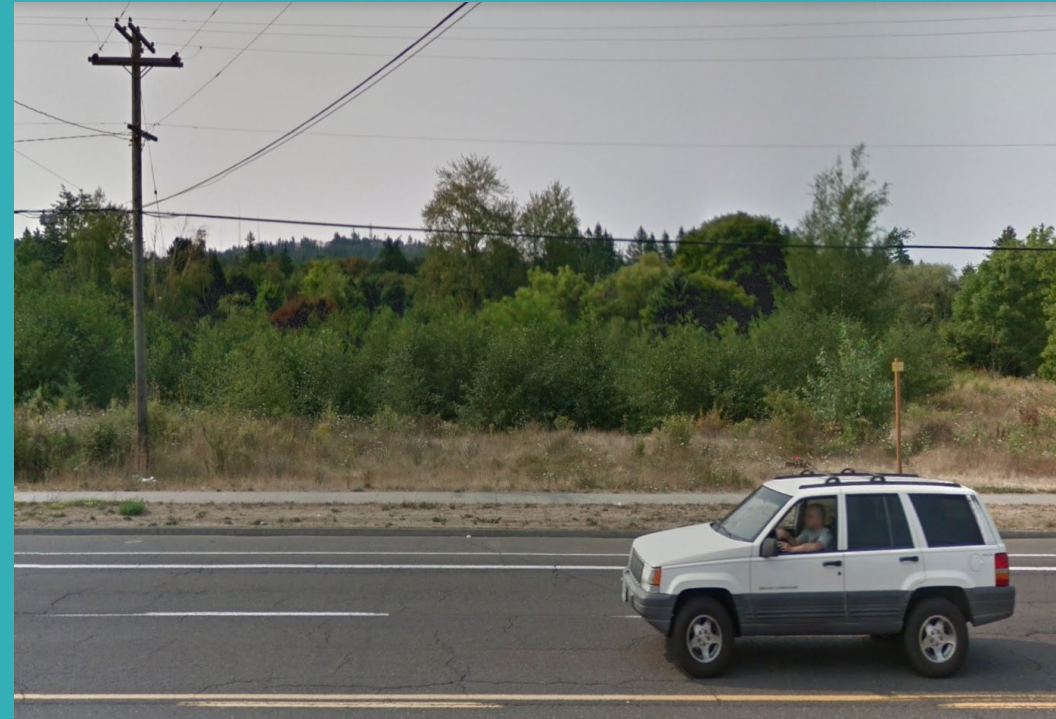
SE 108 th Avenue at SE Foster Road looking south.
