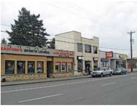
Gateway area commercial buildings
