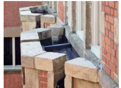
Bay bracing on Trinity Place Apartment building
