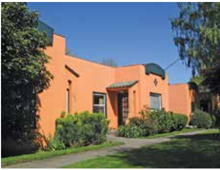
Single-story residential, stucco exterior in Kerns
