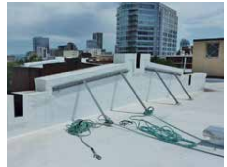
Trinity Place Apartments, parapet bracing
