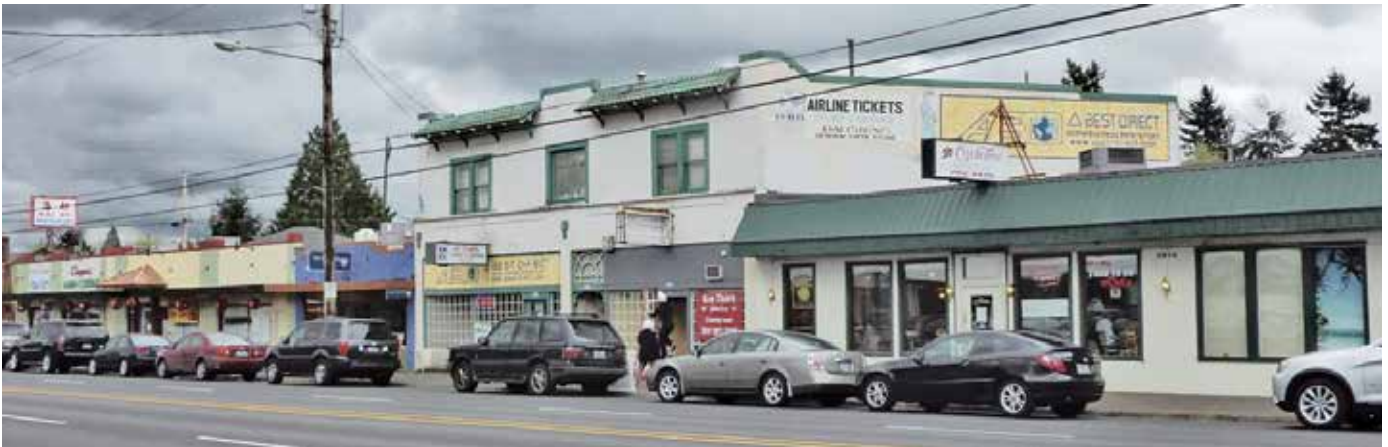
Low-rise buildings have direct exit systems that usually meet current life safety codes.
