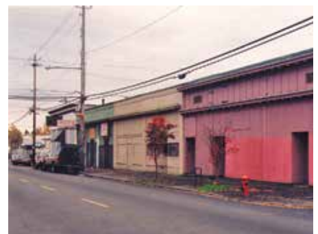
1800 block of NE Alberta Street, 1998, before renovation
