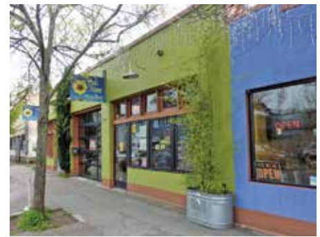
Area 10, NE Alberta Street – King, Concordia Neighborhood – new tenant improvements
