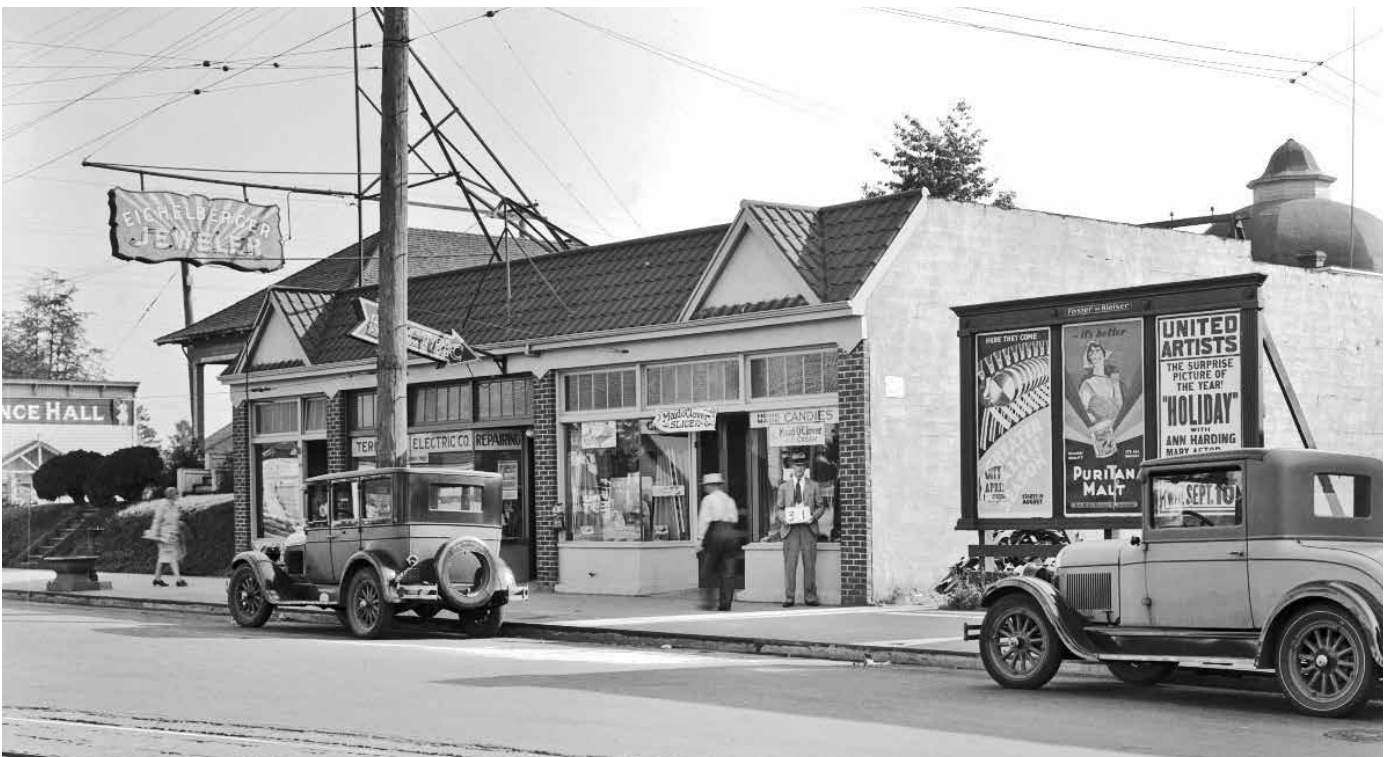
Construction materials include brick, some clay tile, concrete block and board formed concrete. N. Lombard, 1932
