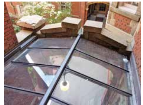
Trinity Place Apartments, entry bracing
