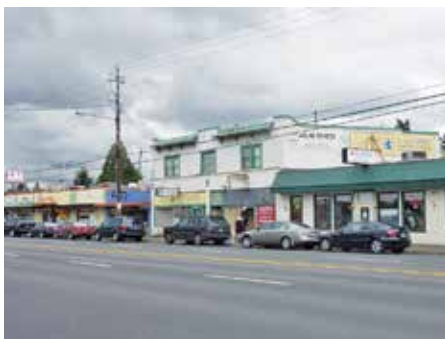
A continuous row of masonry and mixed construction buildings, the differing roof levels can exhibit lateral forces to the intervening walls, but they can also provide some support.
