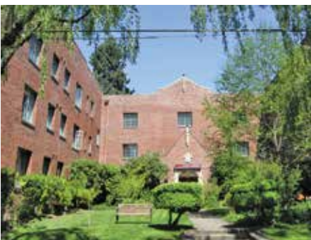
Rasmussen Apartments located within the Kerns Neighborhood, Study area 4
