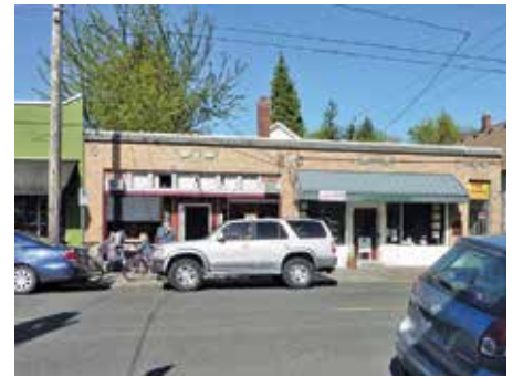
Mixed materials structure
