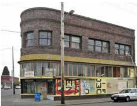
Phoenix Building on SE Foster Road, Study area 1
