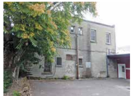
Rear view of the Griessen Building
