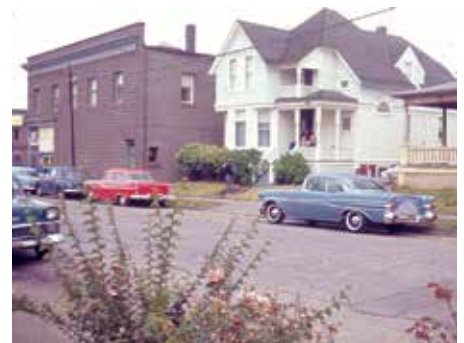
Griessen Building, side and rear, 1964
