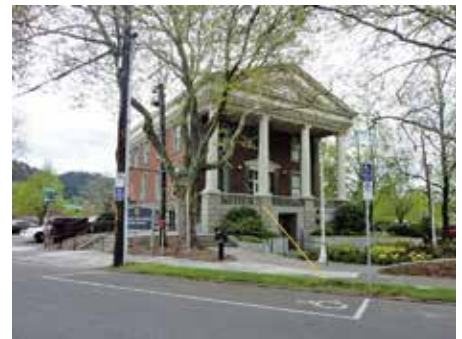
Portland Police Bureau Traffic Division, front view
