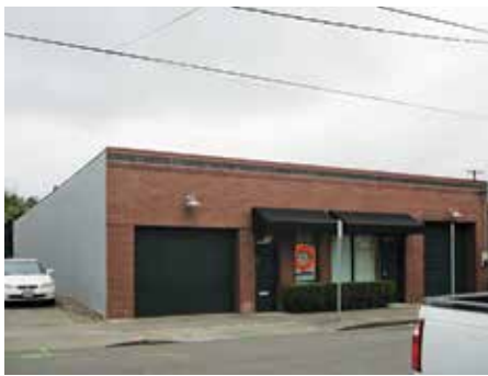
1940s concrete block, low occupancy structure in good condition, likely to have some reinforcement. This indicates a stronger structure with a minimal life safety exposure.
