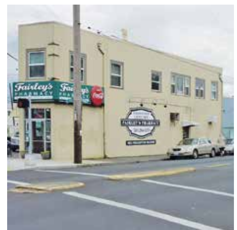
Typical two story building with a single stair exiting to the street, use is different than ground level.
