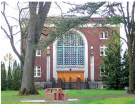
SEIU Building at 6401 SE Foster Road
