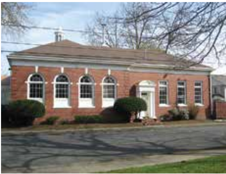
Wickman Building at 4420 SE 64th Avenue
