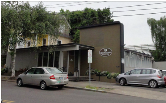
Although just one story in height, this International and Miesian style building (1962) at 1717 SW Madison St. maintains a vertical emphasis.
