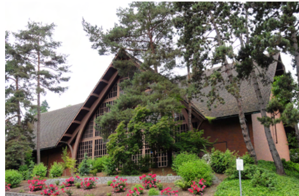
First United Methodist Church (1974) at 1838 SW Jefferson St depicts the Northwest Regional style through its carefully considered relationship with the natural landscape, use of brick and wood materials, and emphasized wood barge board and window details in the center gable.
