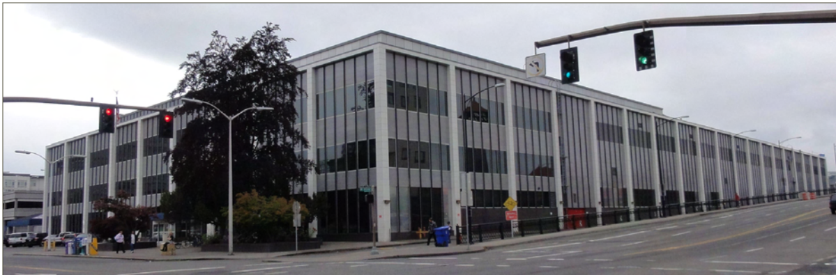
The southeast corner of the United States Post Office and distribution center (1962) at 715 NW Hoyt St, designed in the International and New Formalism styles. This view highlights the business and professional function of the building, while the loading docks for mail distribution are visible from the opposite corner.
