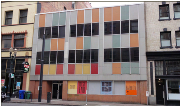
International style office building (1962) at 415 SW 10th Ave uses colorful panels as part of its curtain wall construction.
