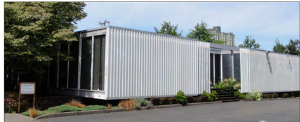
United Metal Trades Association Building (1961) at 906 NE 19th Ave is one of a group of small single-story International style buildings with full-length windows framed by the building's exposed aluminum curtain wall structure.
