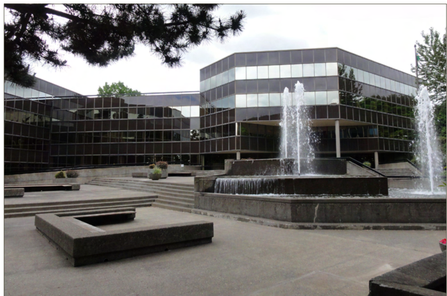
The ADP Plaza building (1982) at 2525 SW 1st Ave is illustrative of the International style with Post-modern influences.
