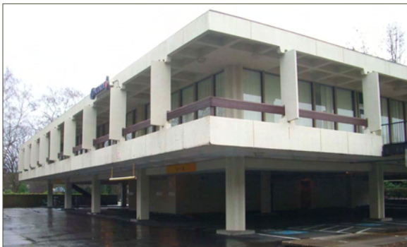
The expansive Lloyd Plaza complex (1965) at 1500 NE Irving St includes three International “piloti” (pier) style buildings that use piers to lift the single-story office to the 2nd floor, allowing ground level parking below.
