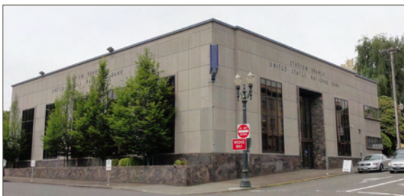
New Formalism style United States National Bank Stadium Branch (1947) at 2000 SW Morrison St, is characterized by its flattened classical details, including the suggestion of pilasters, limited cornice and corner details.
