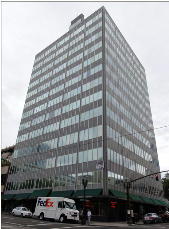
Most high rise commercial buildings, such as the Portland Medical Center (1956) at 505-515 SW 10th Ave, are constructed using a curtain wall structural system that exposes its metal structure, separates gridded windows and metal panels, and displays no ornamentation.
