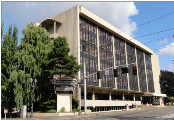
Hotel (1963) at 1021 NE Grand Ave., now operating as the Red Lion Hotel.
