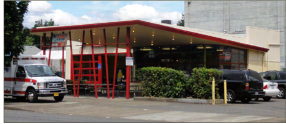
Drive-in restaurant at 438 SE Martin Luther King Blvd is quite expressive of its auto-accommodations. The angled shed roof illustrates the building's Contemporary style.
