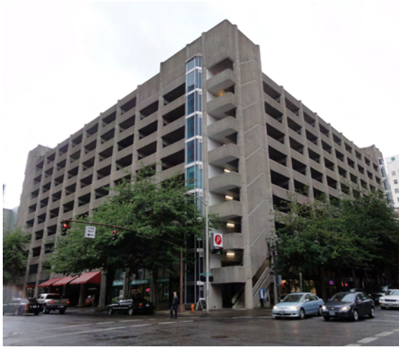
The Brutalism style garage at 1719 SW 6th Ave is characterized by its exposed heavy concrete structure, block-like mass, and repetitive geometric angles.
