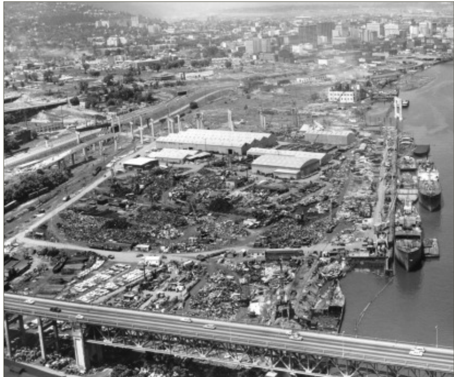
View of South waterfront looking north beyond the Ross Island bridge (1964).
