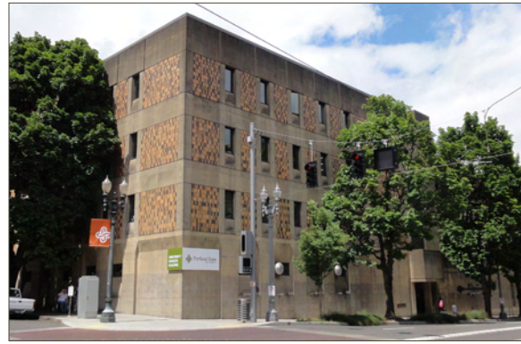
University Services Building (1970) at 617 SW Montgomery St.
