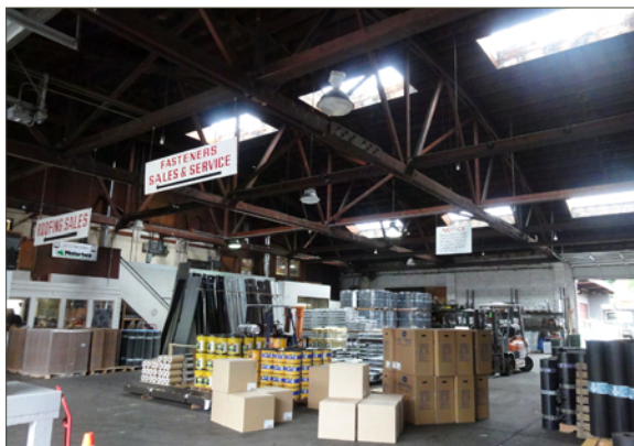
Interior of warehouse (1946/1966) at 1810 SE 10th Ave, which has operated as the Oregon Roofers Supply building since 1963.
