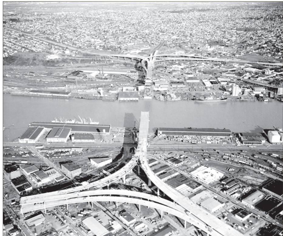
Aerial photo of I-405 and Fremont Bridge construction, view facing east (1971).
