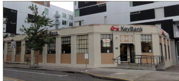
Art-Deco style commercial building (1946) at 1035 NW 14th Ave is characterized by its temple-front features surrounding the corner entrance.
