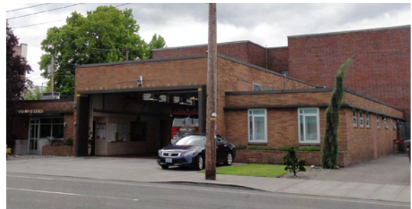
Portland fire Station No. 13 (1955) at 926 NE Weidler St has Ranch style characteristics, including Roman brick large front windows, horizontal massing, and the garage.
