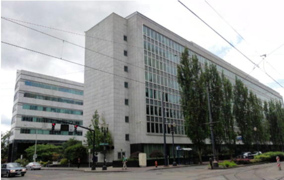
The Bonneville Power Administration building is designed with characteristics of the both International and New Formalism styles, displayed by its cubic form and gridded windows, along with an enframed wall of windows and minimally suggested cornice
