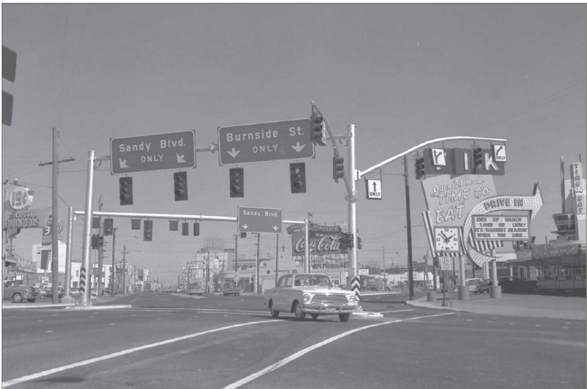
View of Roadside architecture from intersection of E. Burnside St. and NE Sandy Blvd (1965),
