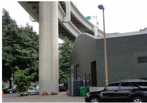
Pillar from I-405 bridge construction required shearing off the southeast corner of this warehouse (1961) at 1516 NW Thurman St.
