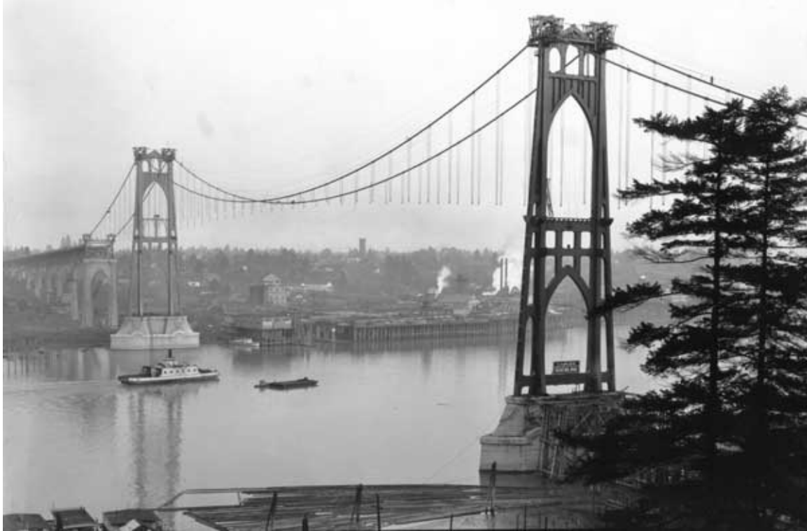
St. Johns Bridge during construction.
