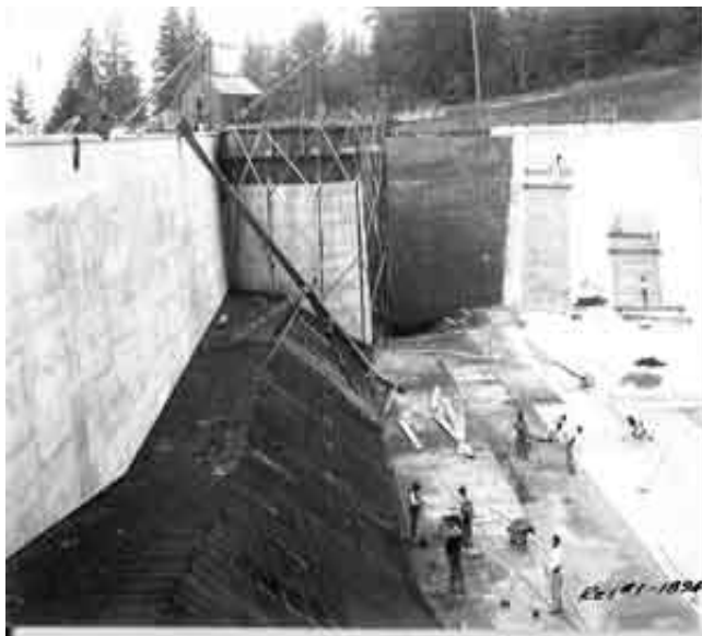
Construction of a reservoir on Mt. Tabor.
