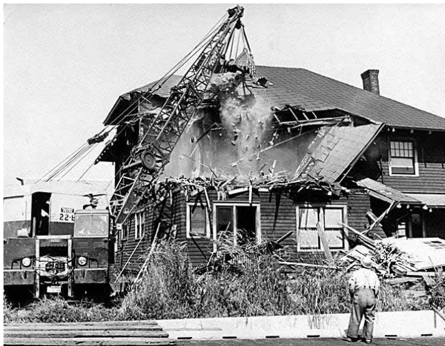
Residential demolition for Lloyd Center.
