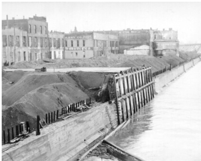
Construction of seawall in downtown Portland.
