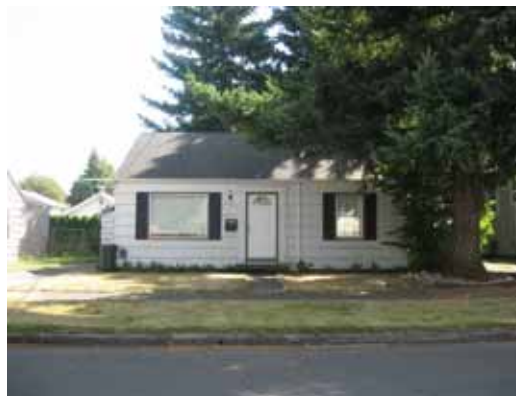
House constructed in 1944, SE 88 th and Alder.
