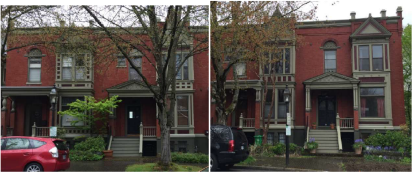
Above: Campbell Town Homes on east half of north side of NW Irving between 17 th and 18 th
