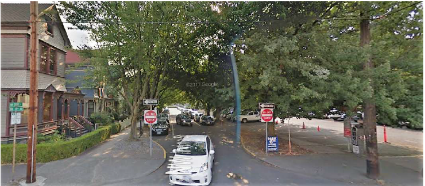
Above: Narrow street opening at NW Irving due to extended curbs, reducing street width at corner to 16 ft; distance curb to curb mid-block is 30 ft per Portland Bureau of Transportation.
