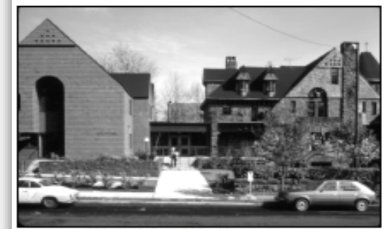
Abbott Hall and MacKenzie House, NW 20 th Avenue and NW Hoyt Street
