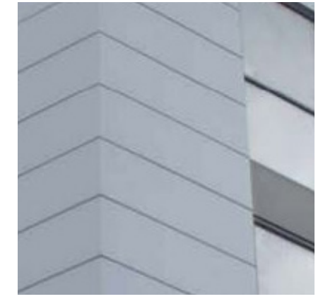
ACM METAL PANELS
