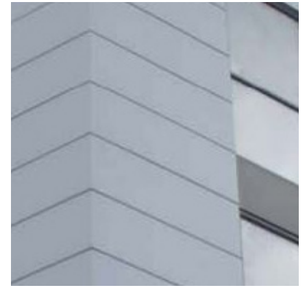
ACM METAL PANELS
