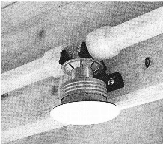
Figure 1-2: ProPEX tee with concealed sprinkler head
