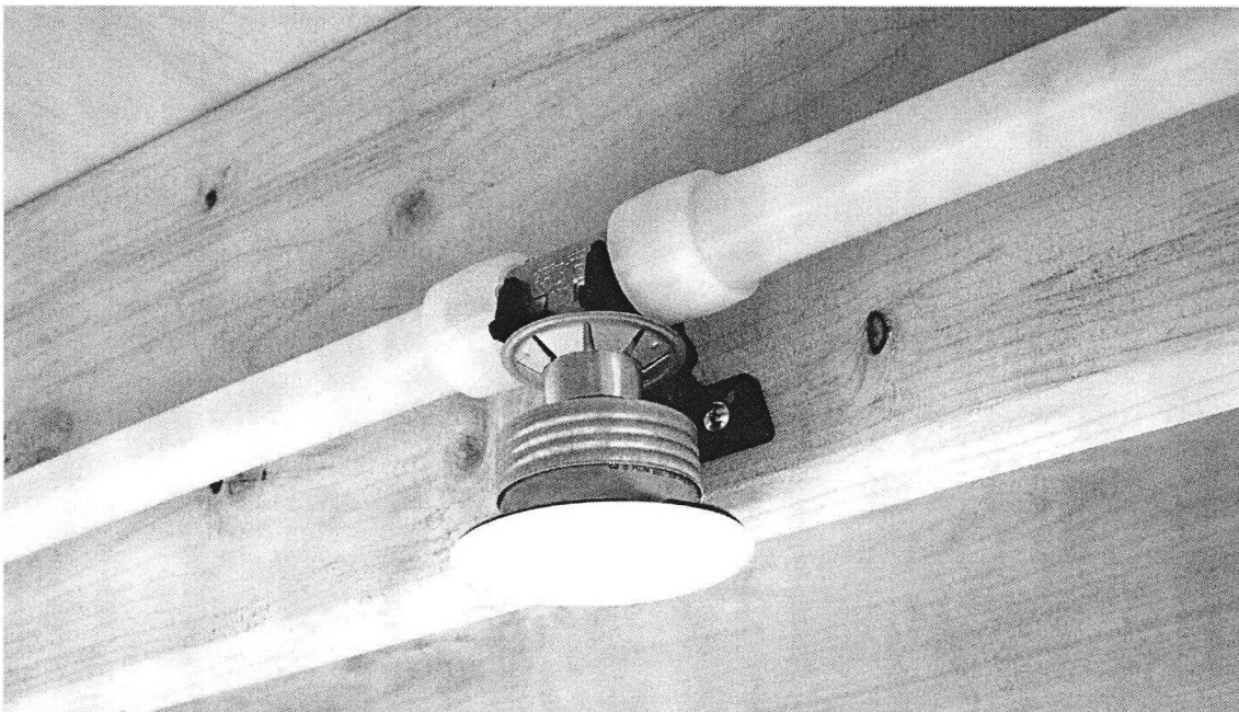
Figure 7-2: Uponor LF brass fire sprinkler adapters
