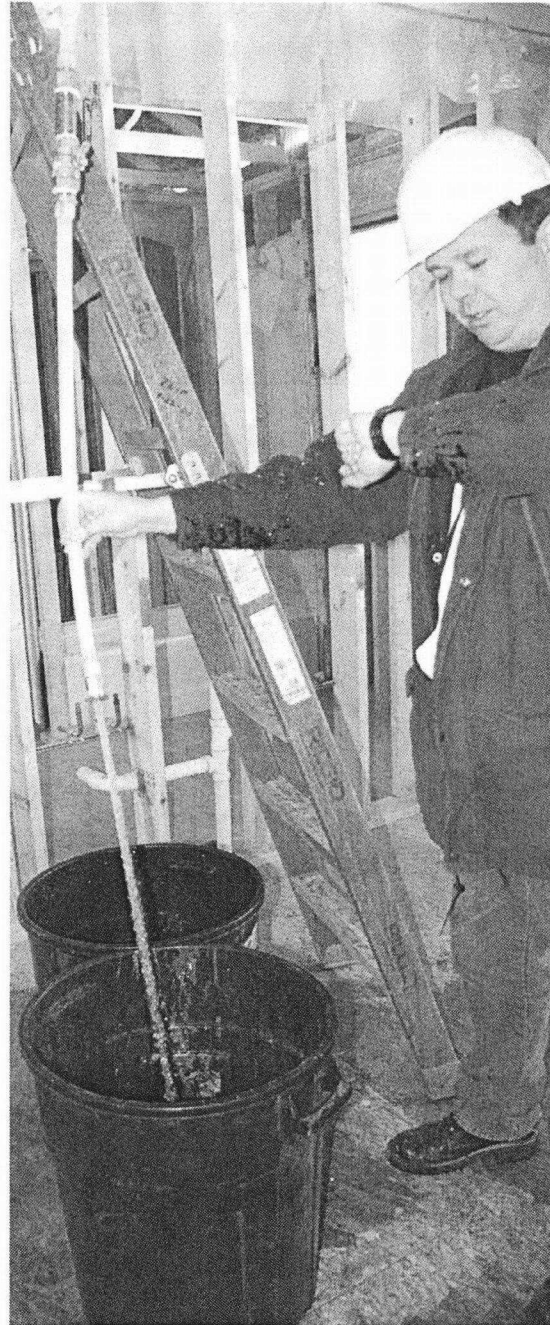
Figure 10-1: AquaSAFE flow test
