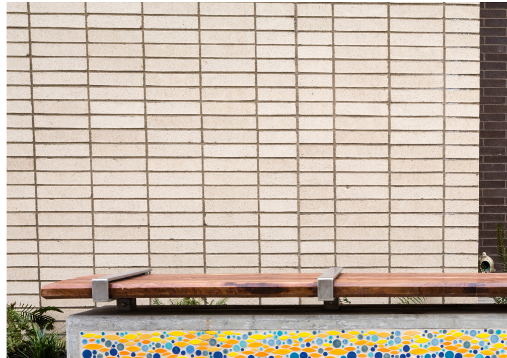
FACE BRICK - VERTICAL STACKED BOND
