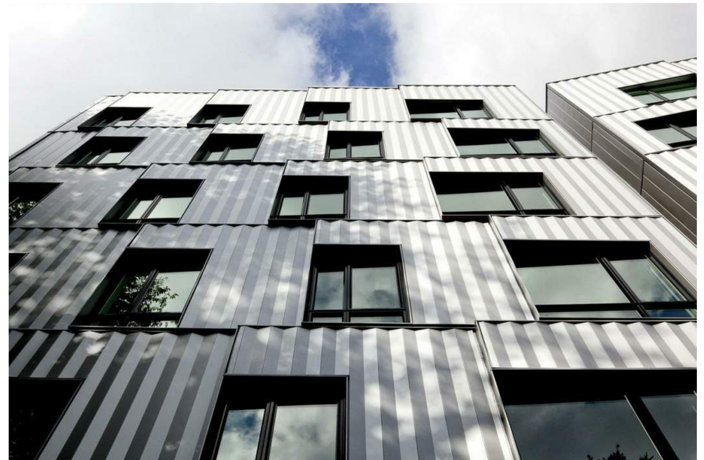
METAL SIDING: TYPE 2 - CHEVRON PATTERN
