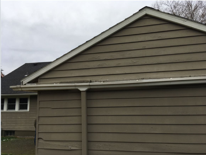
Rear of garage
