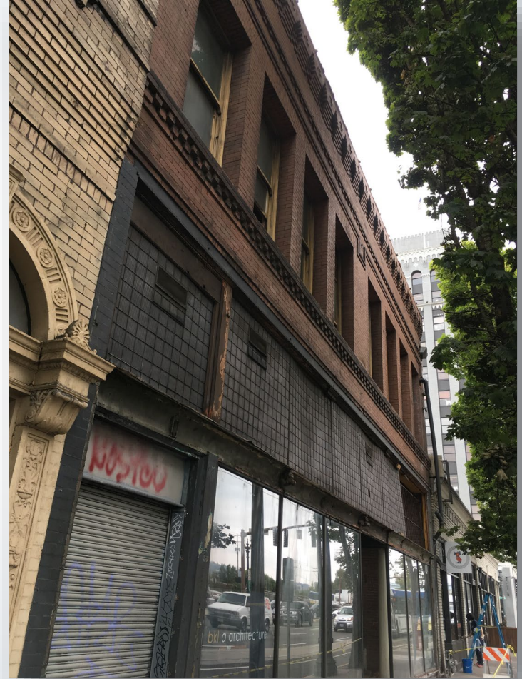
Removal of false façade coverings
