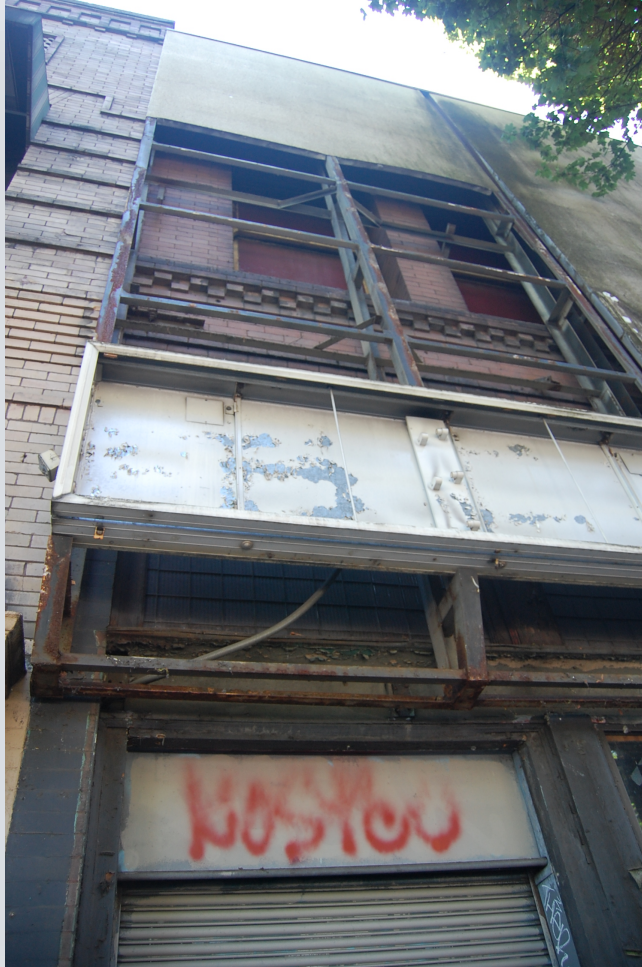
Removal of false façade coverings
