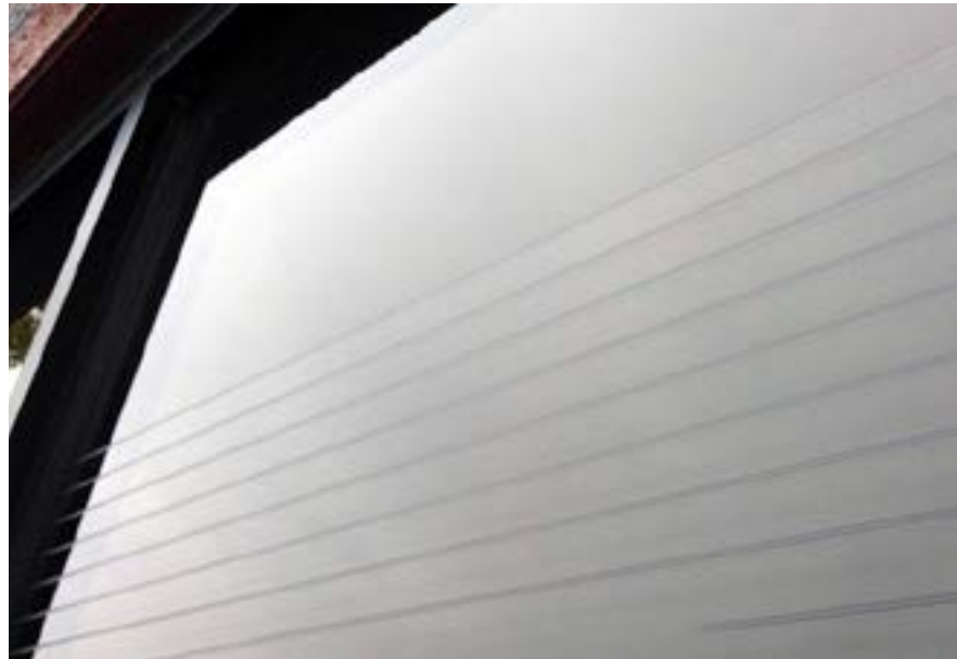
SOLYX Bird Safety Film comes in horizontal and vertical patterns that meet city requirements, but has substantial (~20%) impacts on visual transmission and solar heat gain that are being analyzed.
