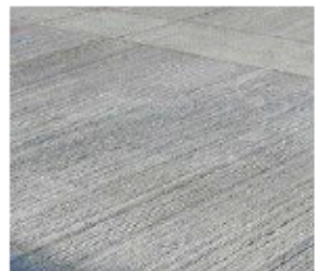
M3. CONCRETE PAVING
