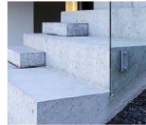
M4. CAST IN PLACE CONCRETE STAIR
