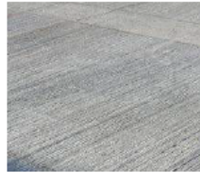
M1. CONCRETE PAVING
