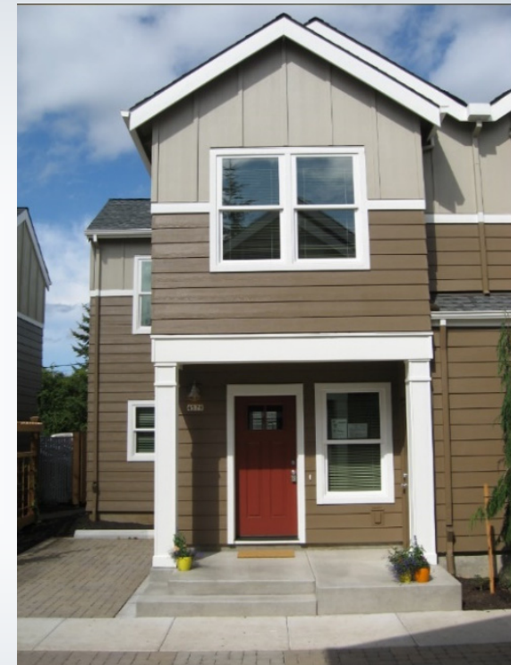
Parking allowed to the side of building front
