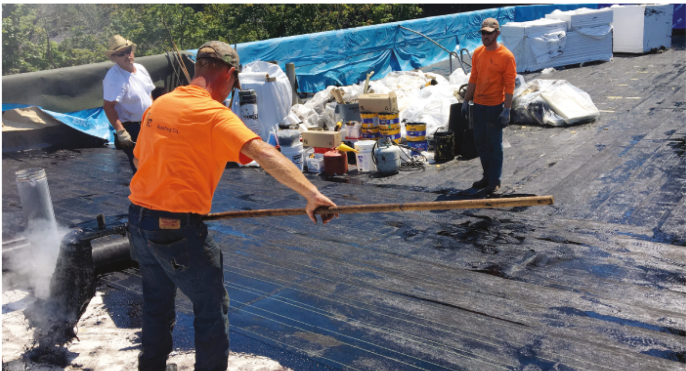
St. Johns Community Center roof construction
