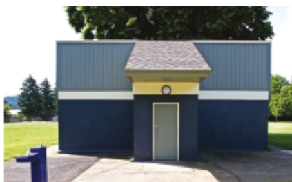
Glenwood Park Restroom (after)
