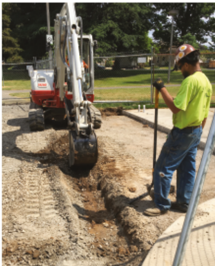
Kenton Park under construction
