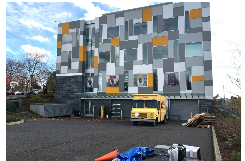
5. View of Loading at Building D
