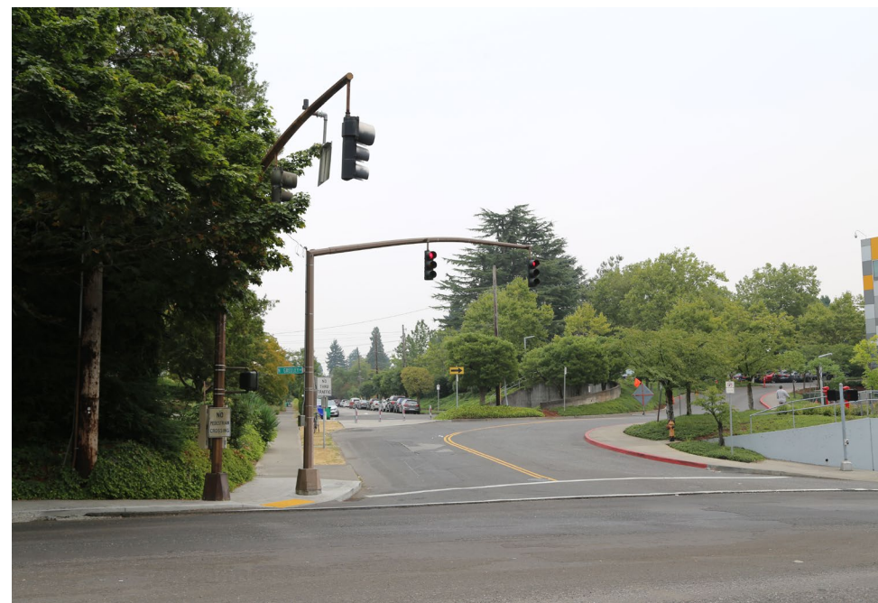
4. View of entry on Greeley @ N. Sumner St.
