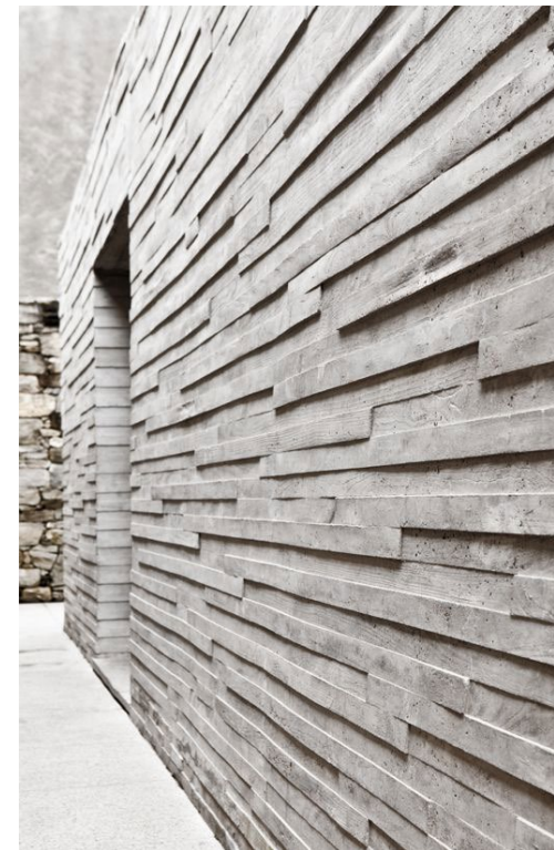
Board Formed Concrete
