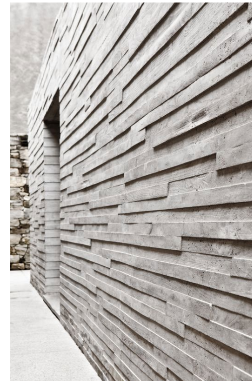
Board Formed Concrete
