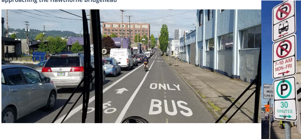
Exhibit 1. Example of Enhanced Transit: Westbound Pro-time Business Access and Transit (BAT) that becomes on-street parking off-peak on SE Madison Street, between SE 10th Avenue and SE Grand approaching the Hawthorne Bridgehead
