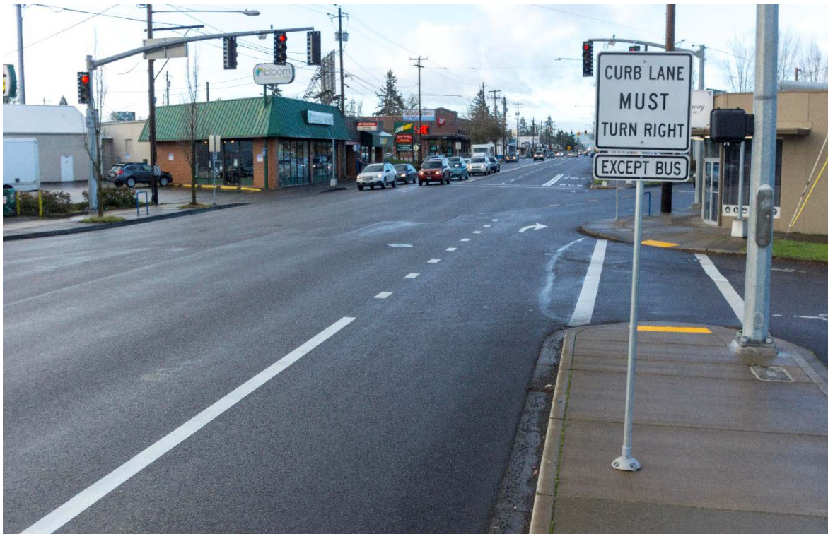
Exhibit 22. Westbound bus queue jump provided on NE Sandy Blvd approaching the signal at 72 nd Ave. This is achieved with a right Turn Only, Except Bus treatments.
