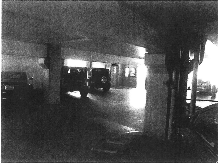
Figure 10, Concrete framing system in the 3 rd floor
