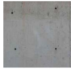
SMOOTH FINISHED CONCRETE
