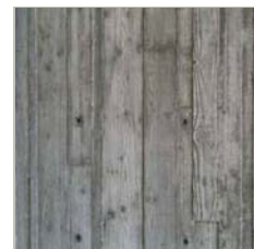
BOARD FORMED CONCRETE
