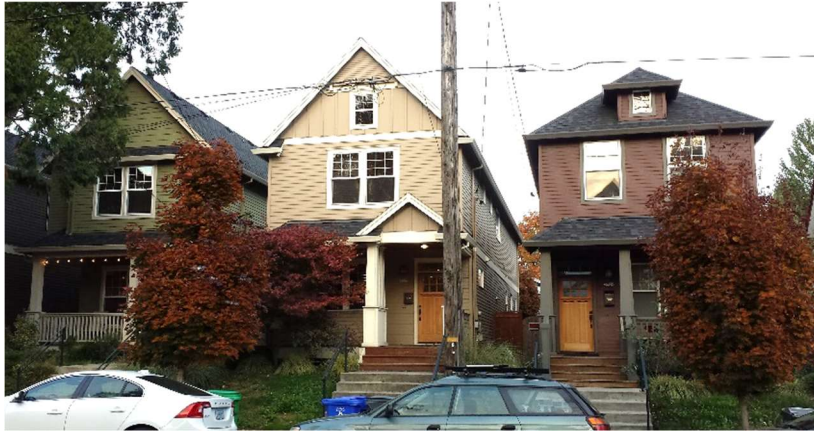
Recently-built narrow lot houses with small side setbacks. The smaller setbacks allow wider houses on 25'-wide lots (19' wide, compared to the 15'-wide “skinny” houses that are built on 25'-wide lots with 5' side setbacks).
