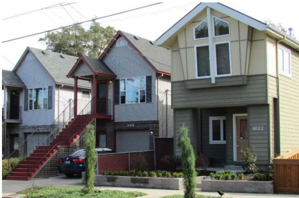
House (center) with long run of stairs that would not meet the distance from grade standard.
