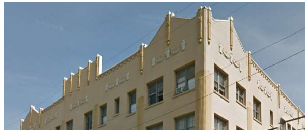
Historic example of parapets providing roofline variety.
