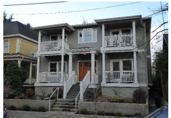
Recent five-plex project with no off-street parking, allowing it to fit into neighborhood context.
