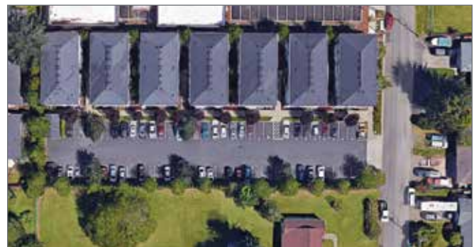
Development on the area's deep lots often leaves little unbuilt or unpaved space.
