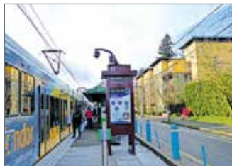
Light rail station at 148th Avenue
