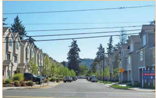
Full street connections are too wide to fit into many lots in Eastern neighborhoods (50 foot wide street shown).
