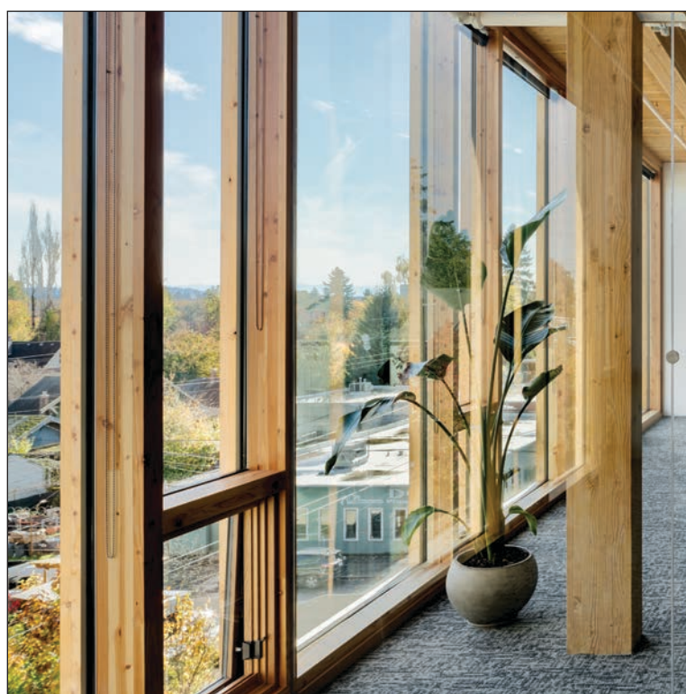
Wood window system from interior
