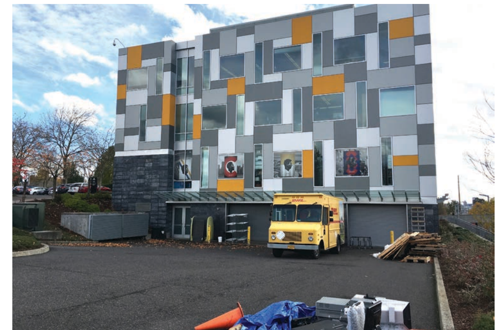
5. View of Loading at Building D
