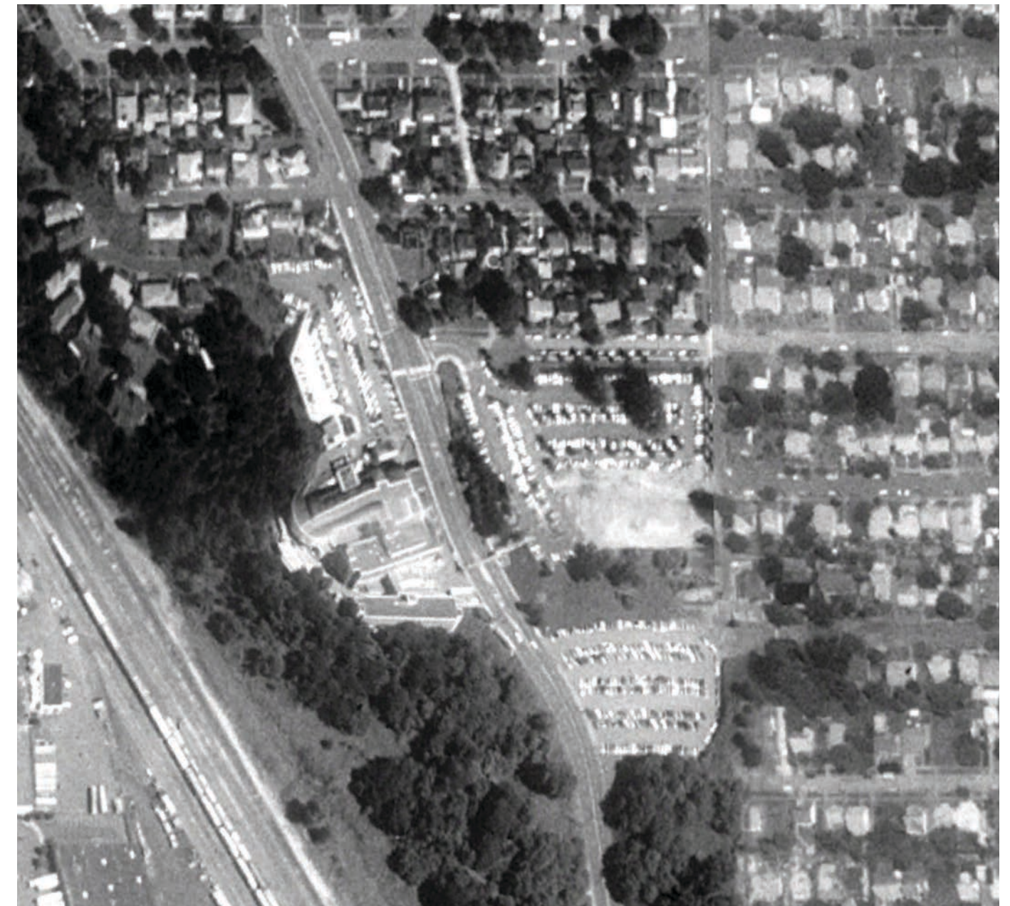
Bess Kaiser Hospital site aerial, 1990. Surface parking lots define the area between Greeley Ave, Sumner St, and Delaware Ave
