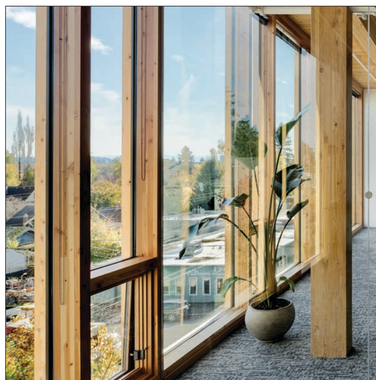
Wood window system from interior
