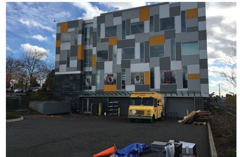
5. View of Loading at Building D
