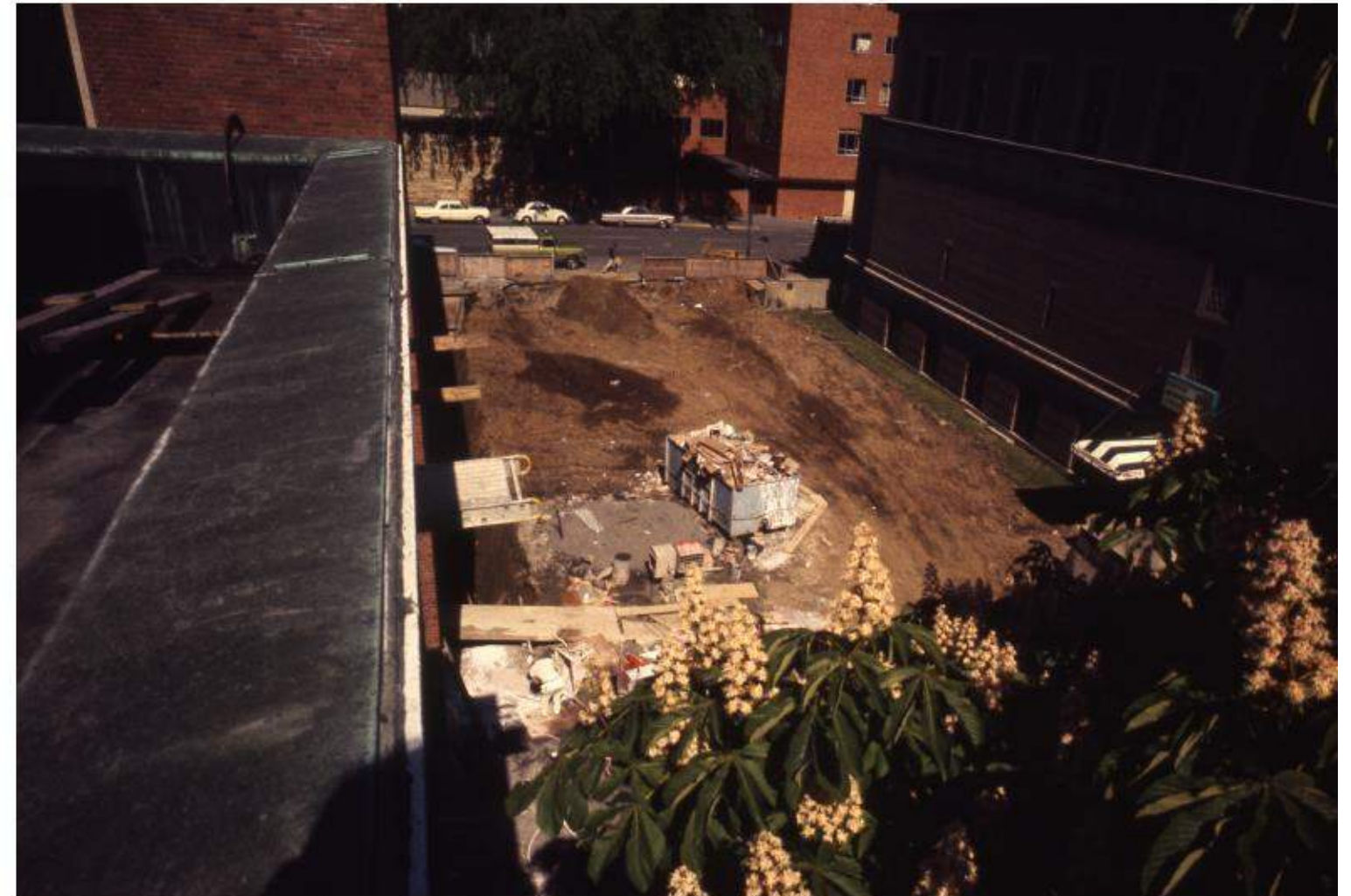
Construction of sculpture court - Madison Street facing 10 th Ave. ca. 1969
