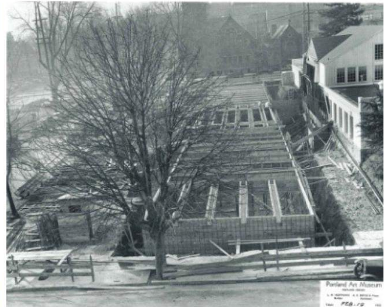
Construction of Ayer Wing, 1932 Facing south from Madison toward Jefferson
