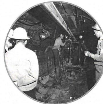
City of Portland Archives A2001-007.80 Sewer tunnel connecting Tryon Creek Sewage Treatment Plant under construction.
