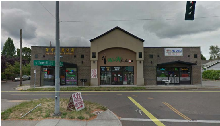
Commercial block construction at
