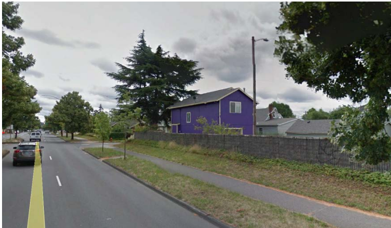
Concrete wall on south side and 2
