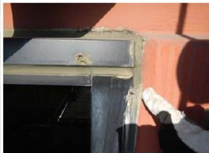
Sealant applied under head flashing
