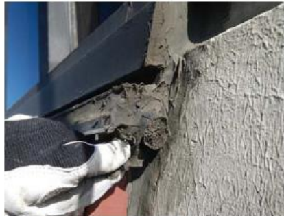
Multiple layers of sealant applications
