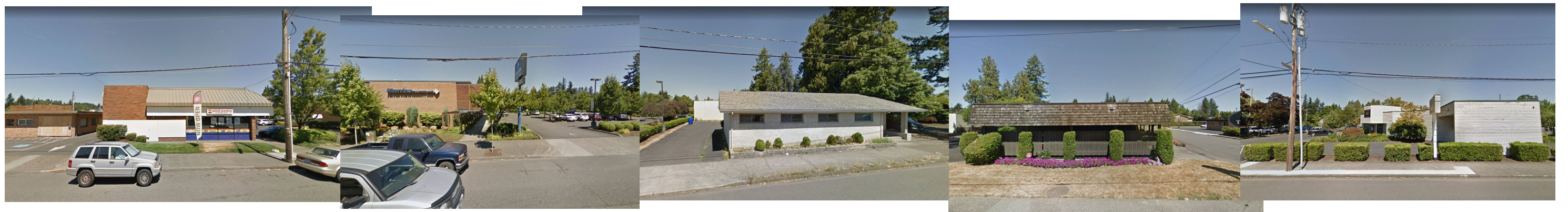
HALSEY STREET - NORTH SIDE
