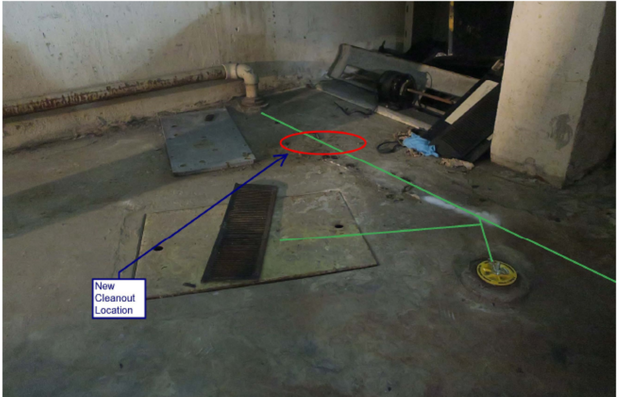
Figure 6: New cleanout location
