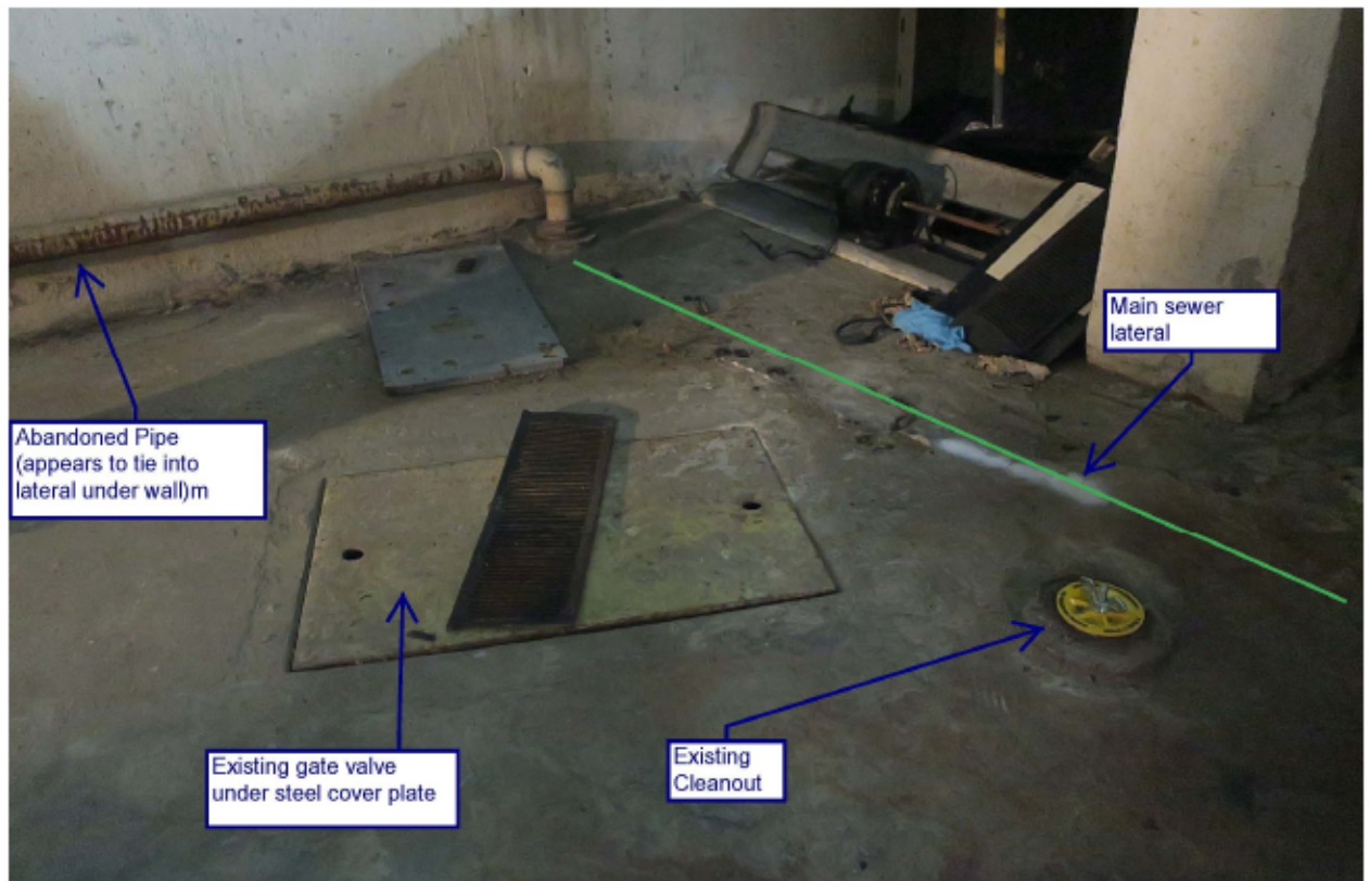
Figure 4: Cleanout and abandoned pipe in crawl space
