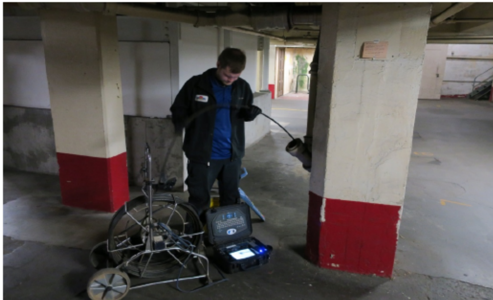
Figure 2: Apollo Plumbing performing sewer camera work
