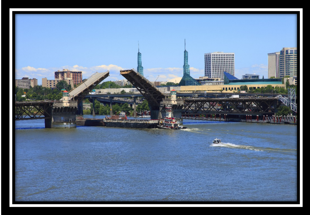
Working draw bridge
