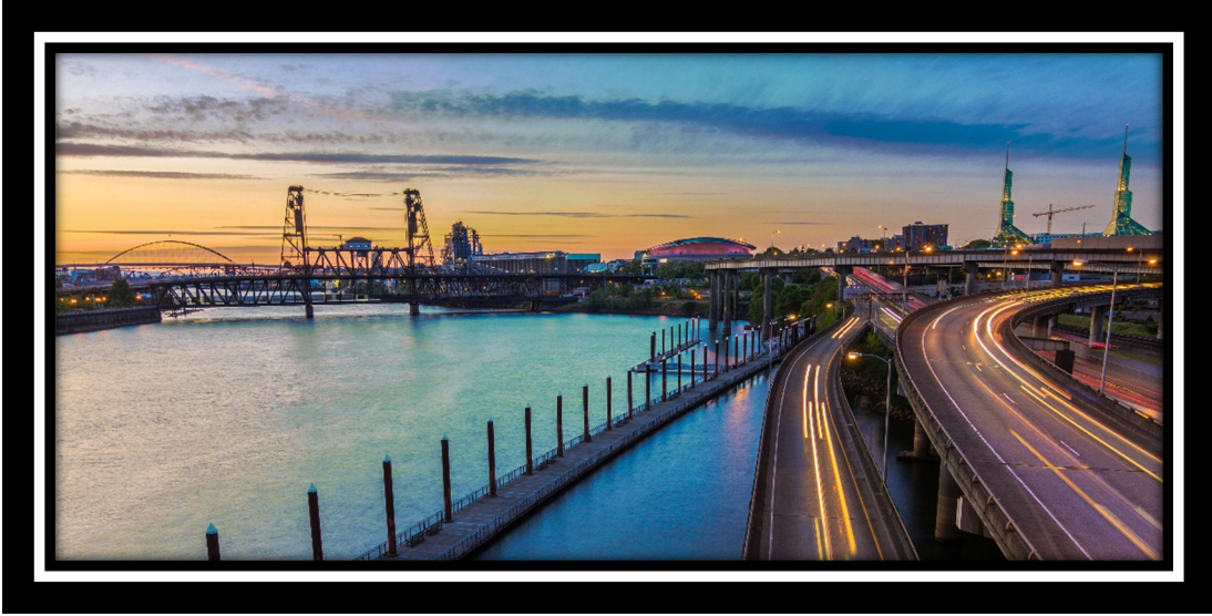
Freeway lights, Moda Center, Convention Center
