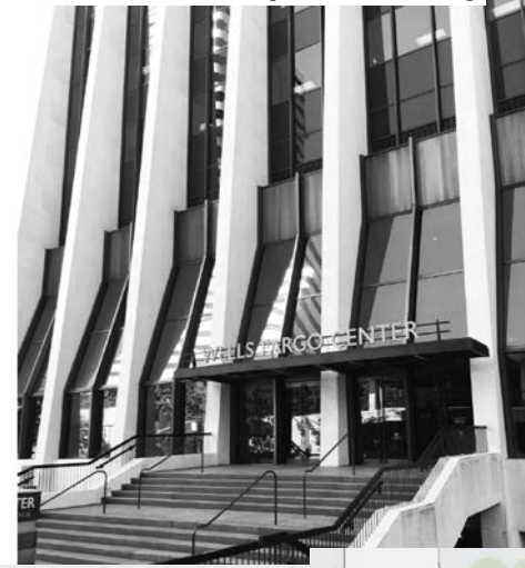
Tower Entry Existing
