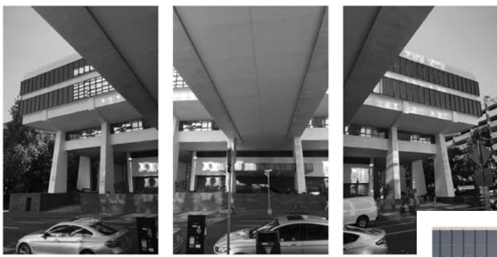
Existing Data Processing Building
