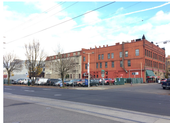
View of SE MLK Looking Northeast
