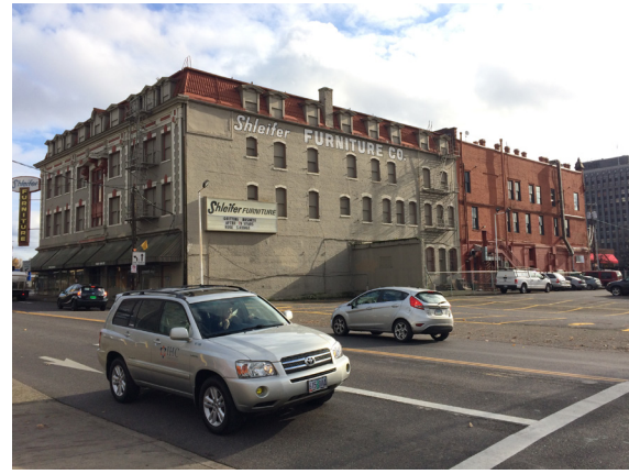
View of SE Stark Looking Southeast
