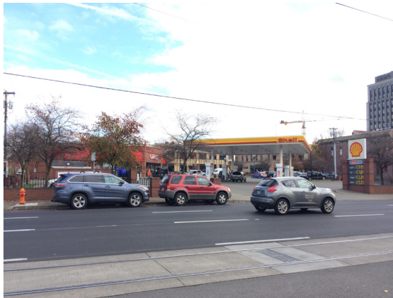
View of SE MLK Looking Southeast
