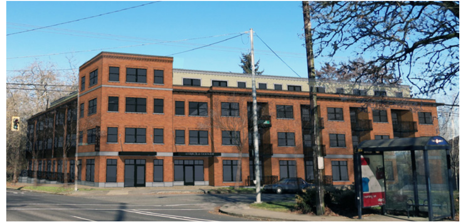
DAR II - 3-STORY 'L'-SHAPED BUILDING WITH 4-STORY TOWER & PENTHOUSE
