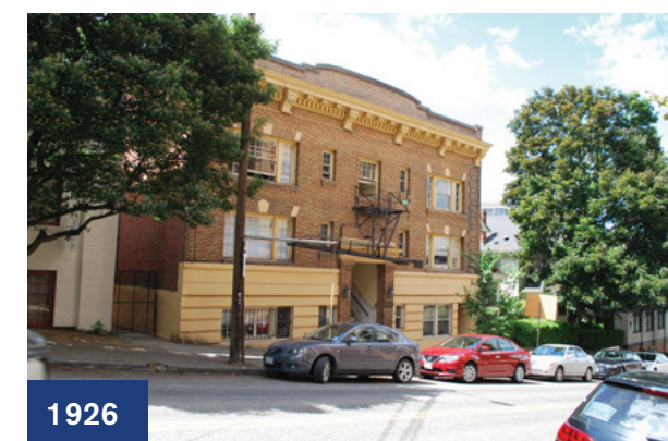
YELLOW BRICK CORNICE DENTILS RUSTICATED BASE
