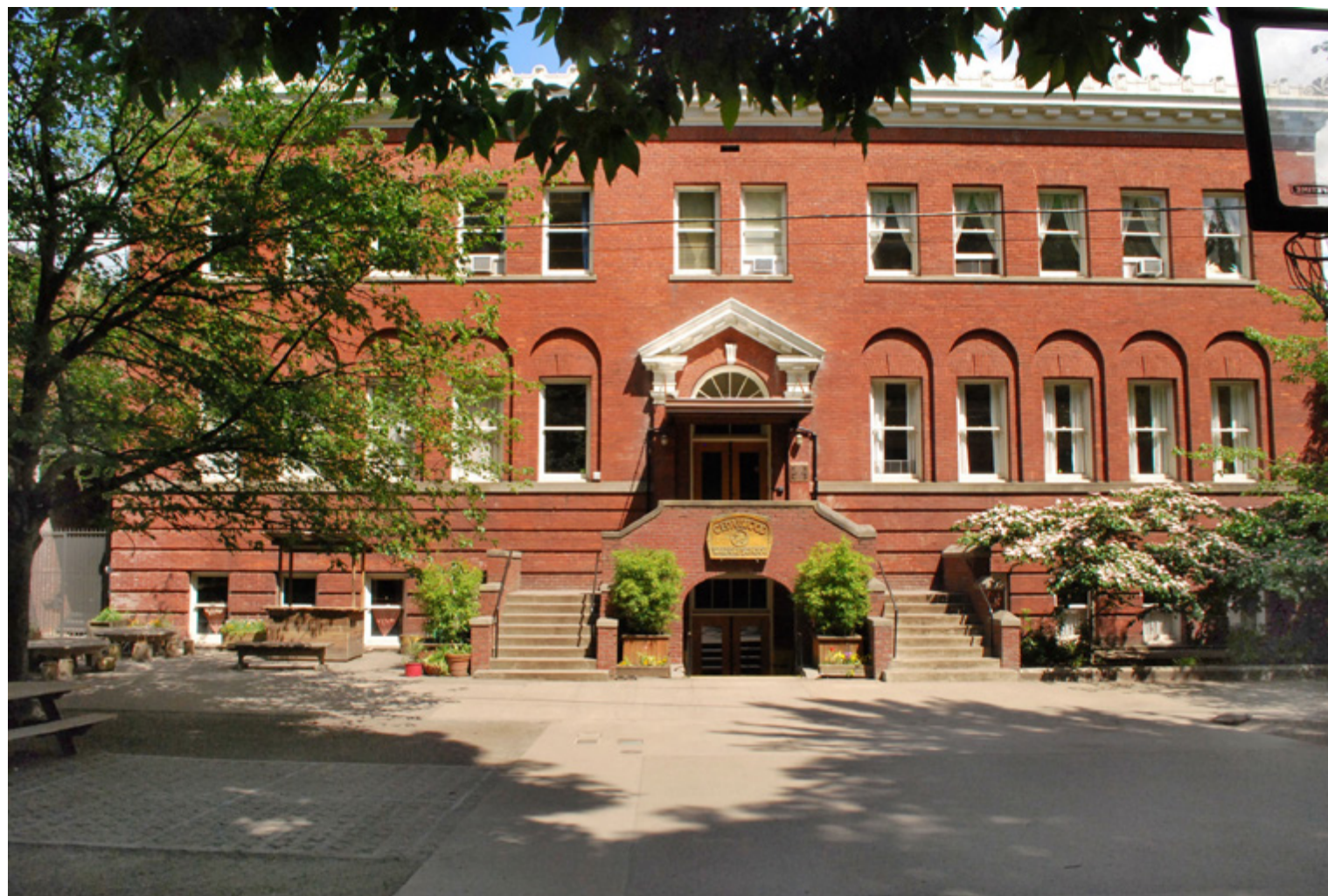
NEIGHBORHOOD HOUSE 3030 SW 2ND AVENUE 1910
