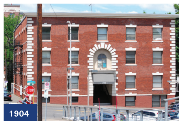
RED BRICK CORNICE QUOINS KEYSTONES
