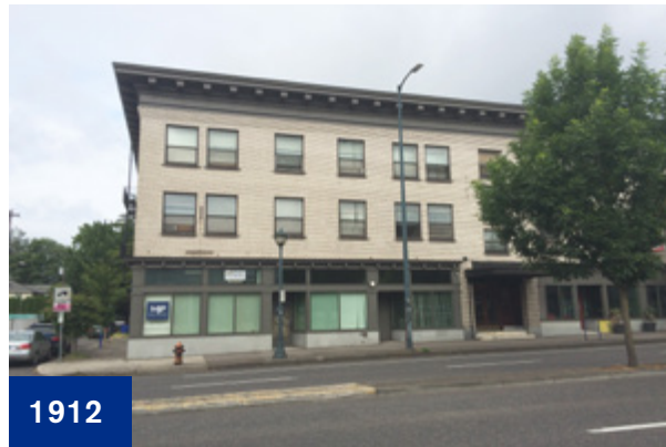
CREAM BRICK CORNICE DENTILS
