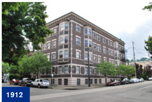
BROWN BRICK CORNICE DENTILS ORIEL BAYS RUSTICATED BASE QUOINS
