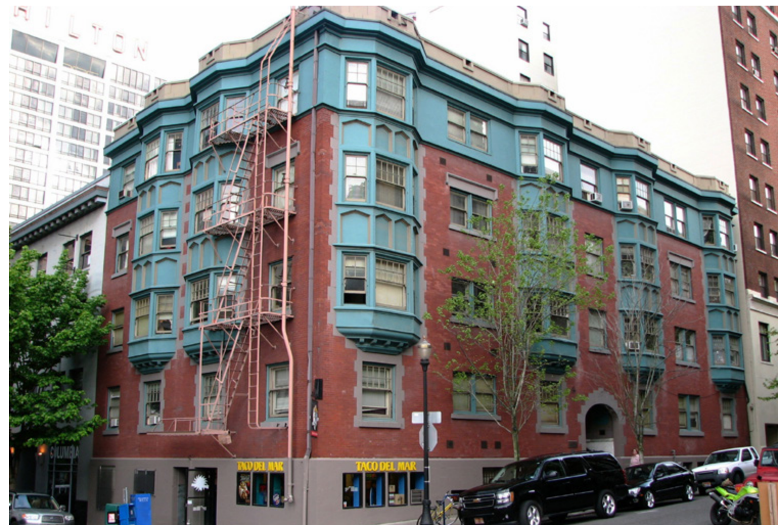
THE ADMIRAL APARTMENTS 910 SW PARK AVENUE 1909
