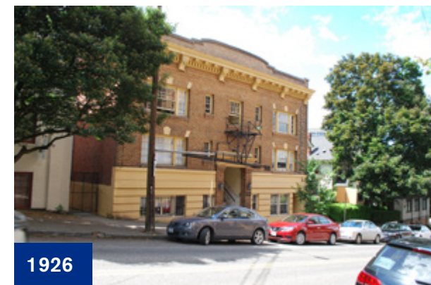
YELLOW BRICK CORNICE DENTILS RUSTICATED BASE
