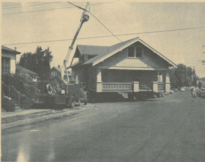
Structure being moved into the project at 3704 North Gantenbein by Mr. C. F. Phillips, Owner.
