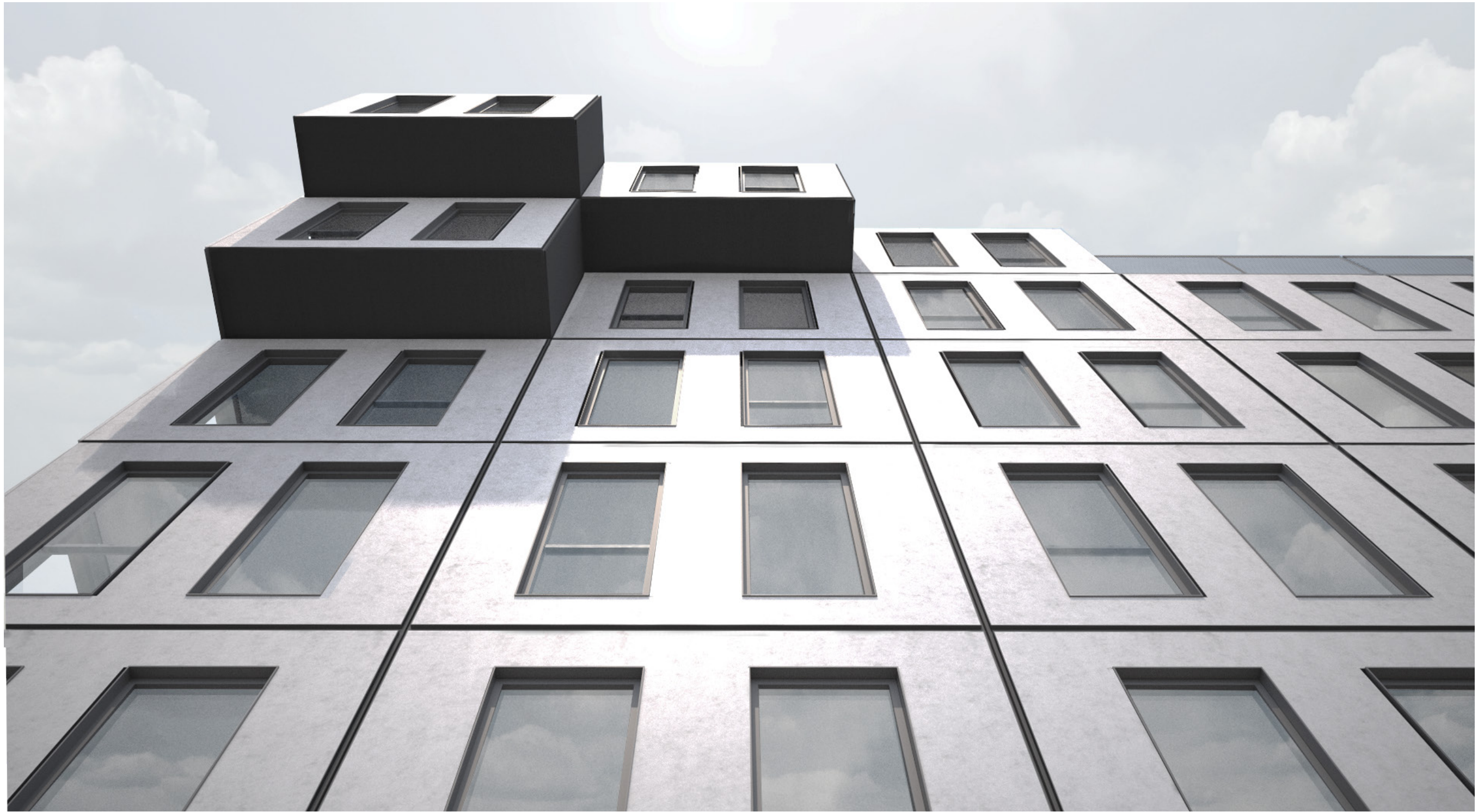
VIEW FROM COURTYARD
