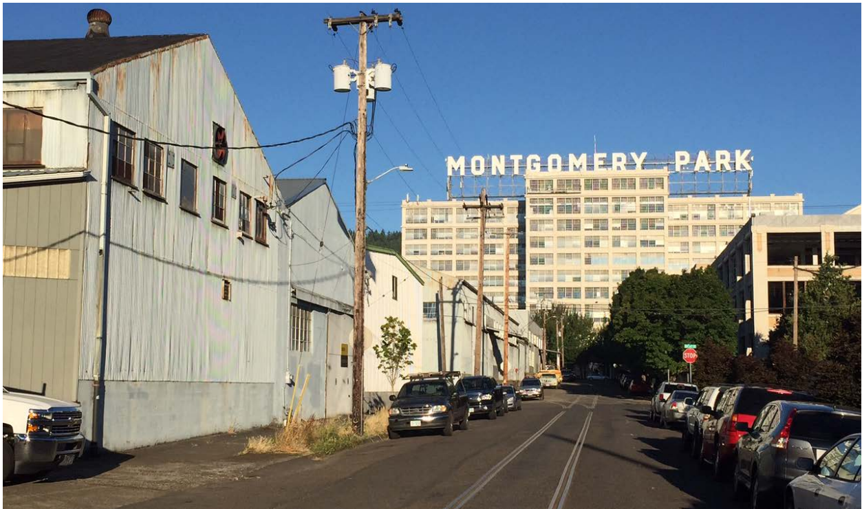
EG2 General Employment zoning is recommended at the Montgomery Park office building.
