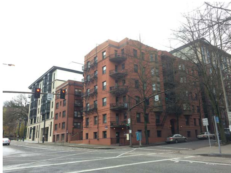
EXISTING TIFFANY AND CLAY APARTMENTS
