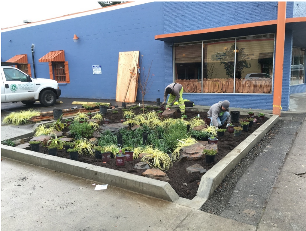
Figure 22 FY 2017 Example Retrofit #2
