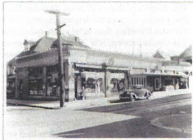
Looking southeast at 622 NW 23rd Avenue
