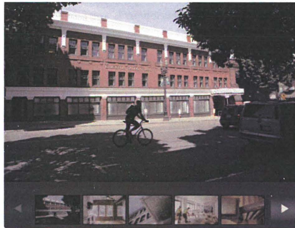
The facade facing NW 2nd Avenue just north of Burnside. Innovative Housing has remodeled two Old Town buildings into 62 studio and one-bedroom apartments. 52 of which are affordable housing. Salvaged material and original features from the Erickson Saloon and Fritz Hotel Buildings, built in 1912, were retained for use throughout the new
