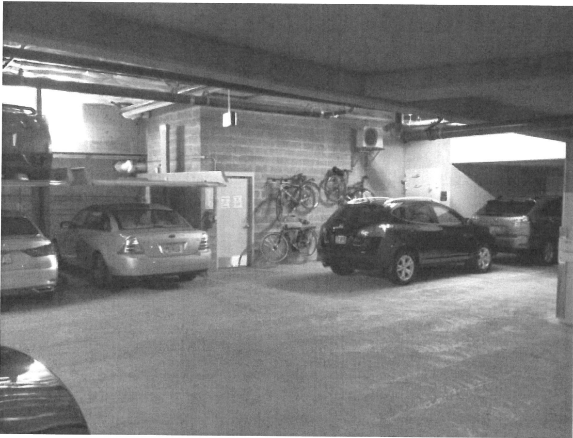
Lifts and tandem parking at The Strand condominiums in Portland. Photo by Ari Ronai-Durning.
