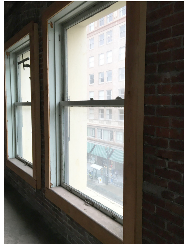
EXISTING DOUBLE-HUNG WINDOW
