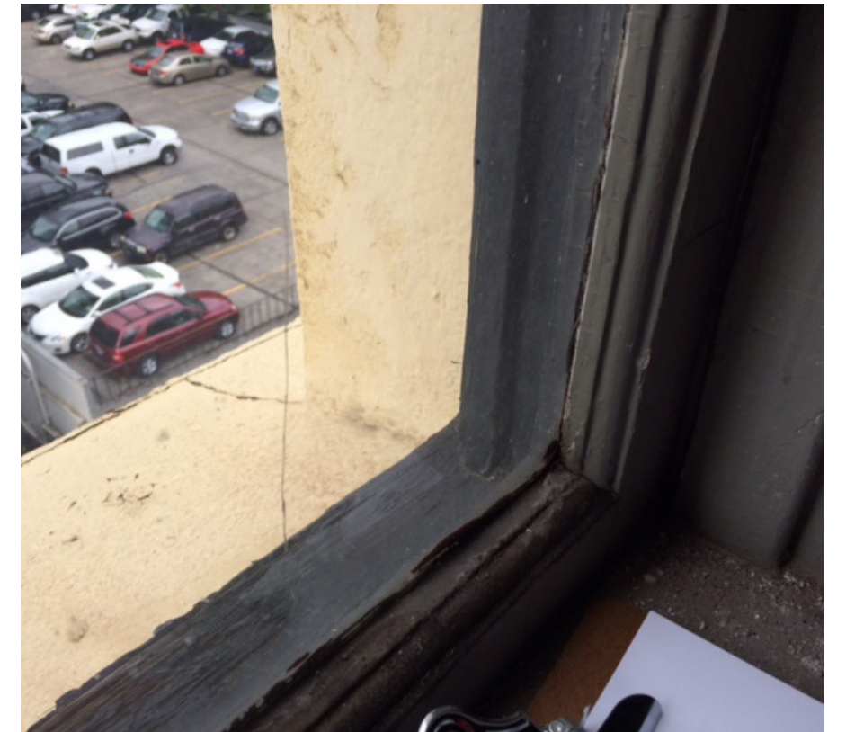
EXISTING DOUBLE-HUNG WINDOW
