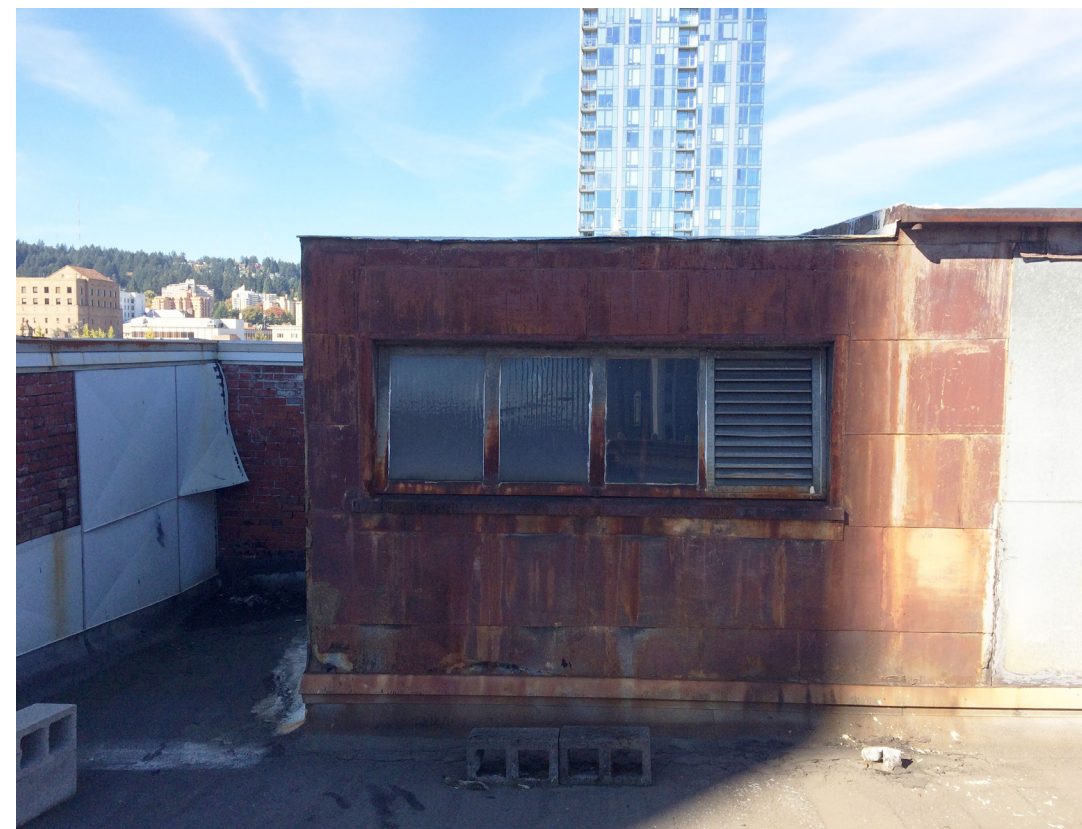
EXISTING STAIR PENTHOUSE & SOUTH BUILDING PARAPET
