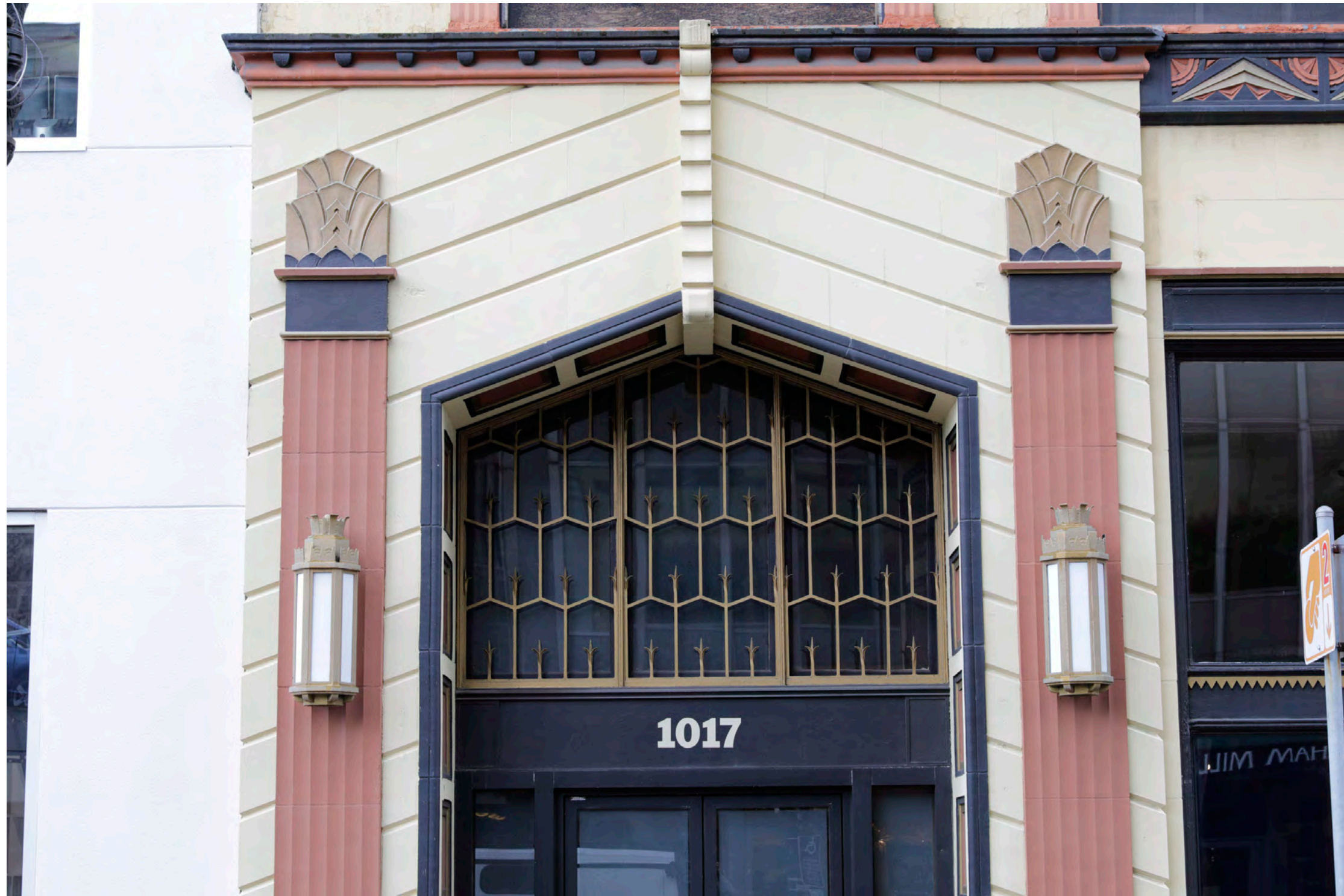
EXISTING SOUTH LOBBY ENTRANCE
