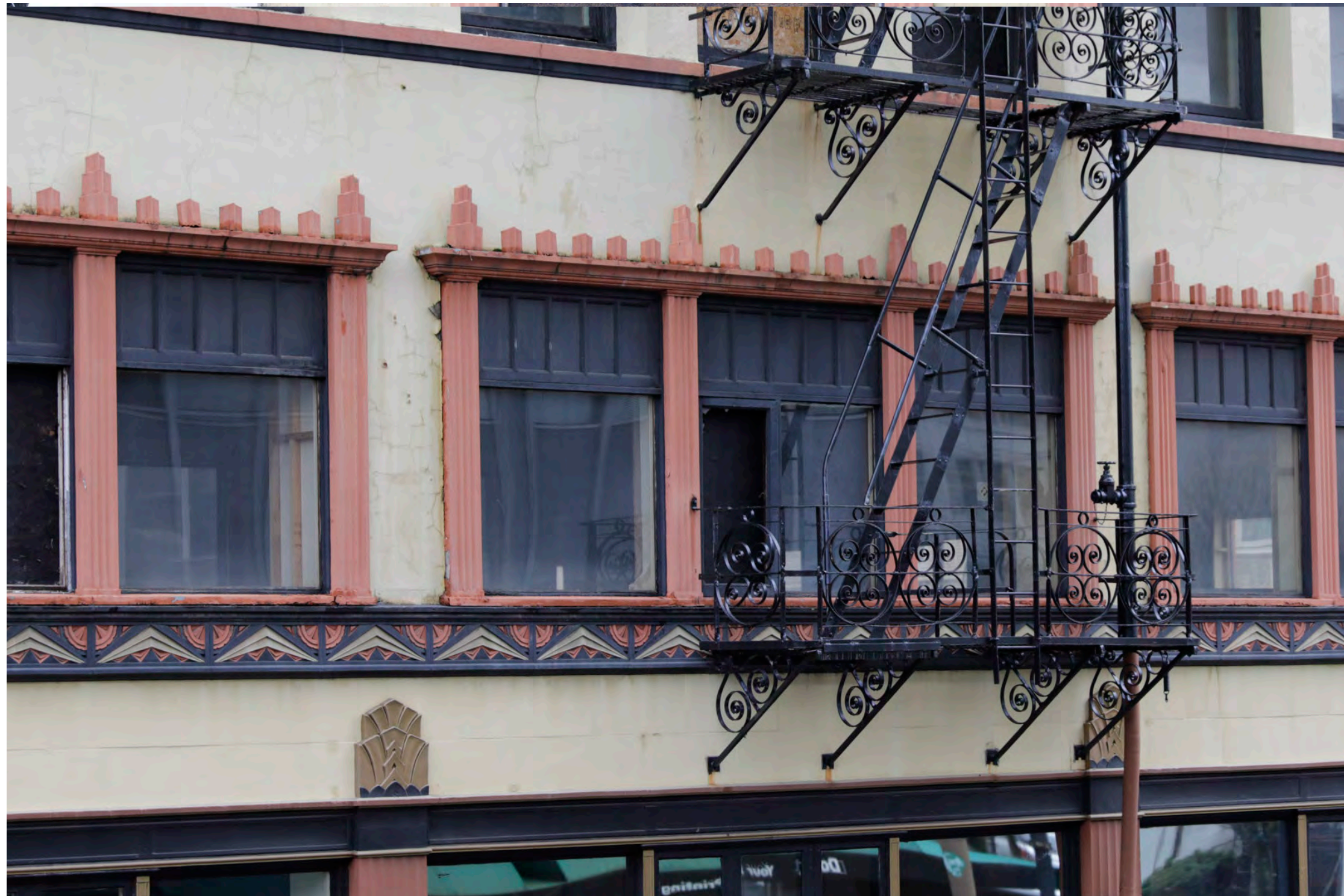
EXISTING STUCCO, TERRACOTTA AND WINDOWS
