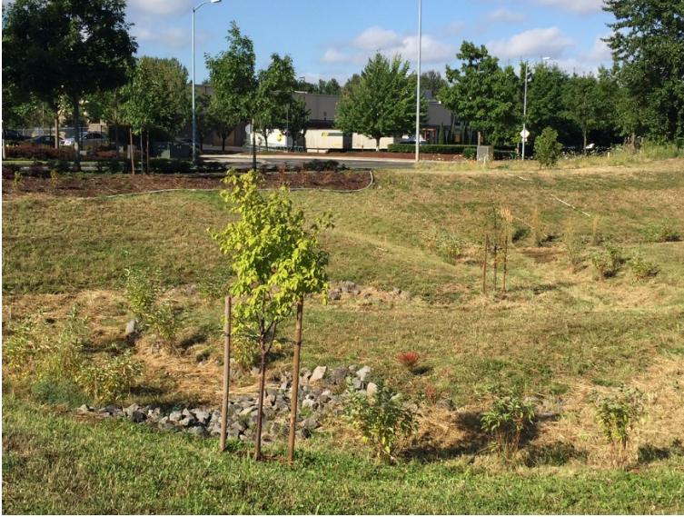
Wide swales, native landscaping, and downward-shining exterior lighting can improve stormwater and habitat functions, like shown here on industrial sites near PDX Airport.
