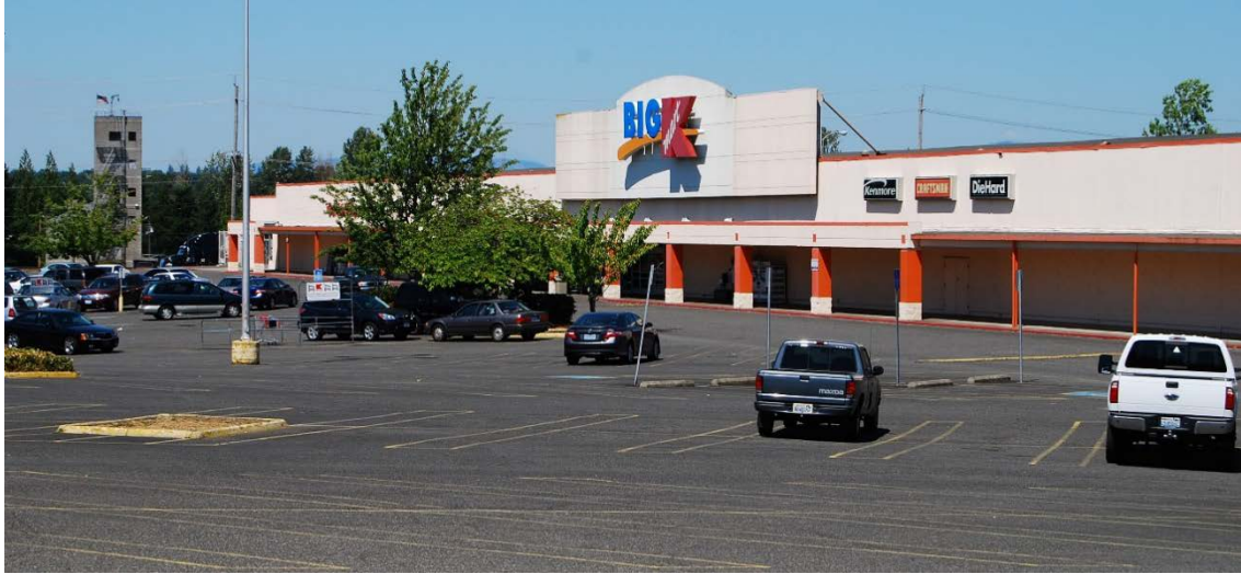
EG2 General Employment zoning is recommended at the Kmart/Sears site at NE 122 nd and Sandy.
