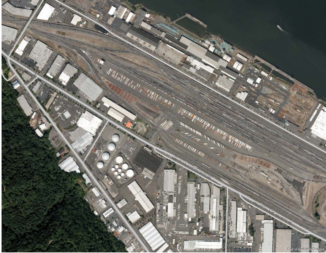
Typical land use patterns in the Prime Industrial overlay zones consist of large-scale industry served by a mix of railroad, harbor, airport, or truck infrastructure, such as in the Northwest Industrial District shown here.
