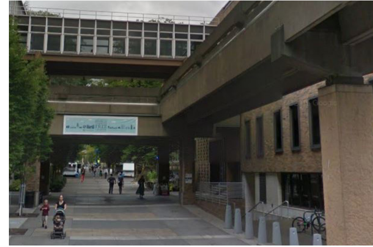
SW HARRISON ST PEDESTRIAN BRIDGES FACING WEST
