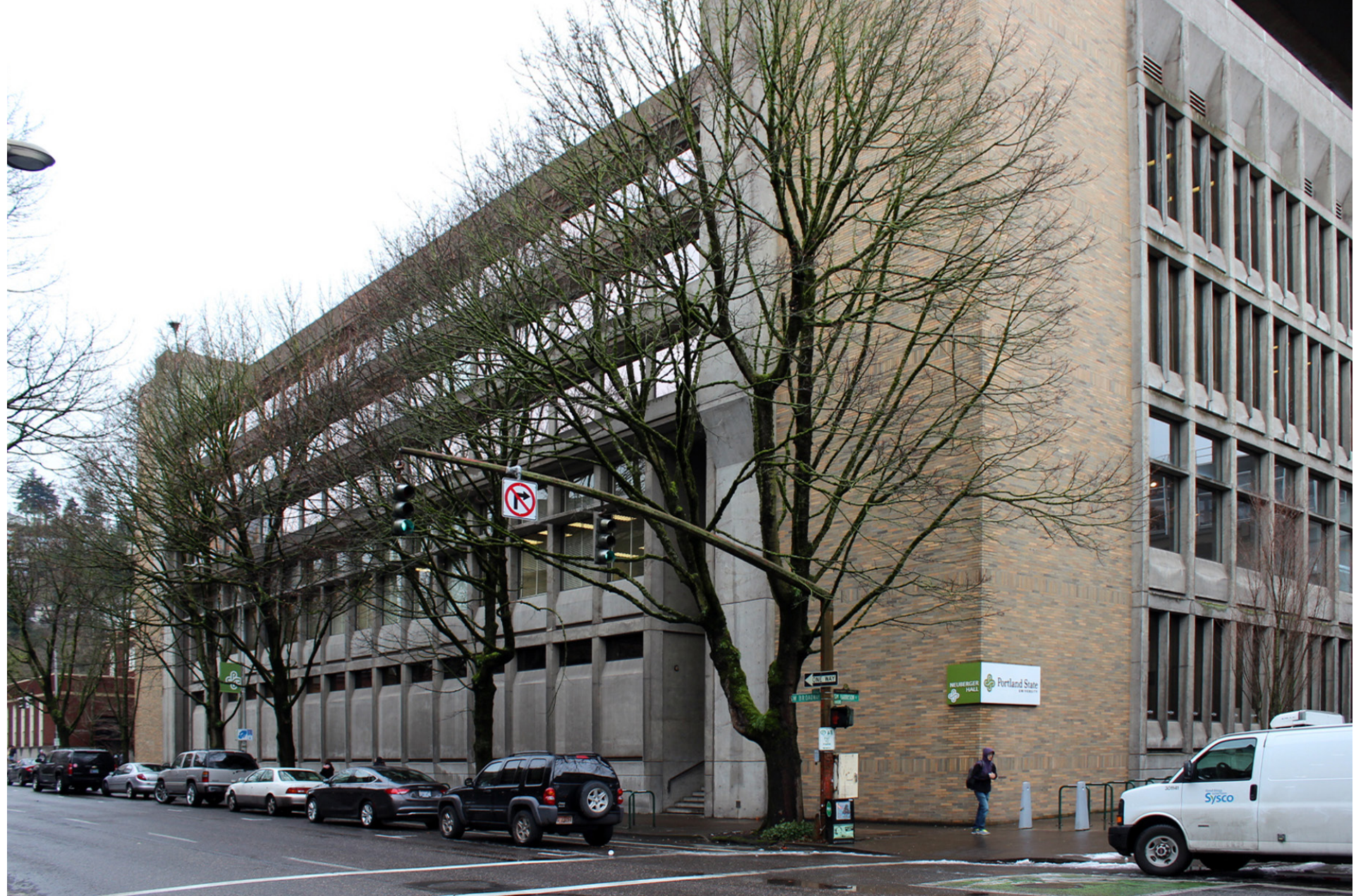
EXISTING NORTHEAST CORNER
