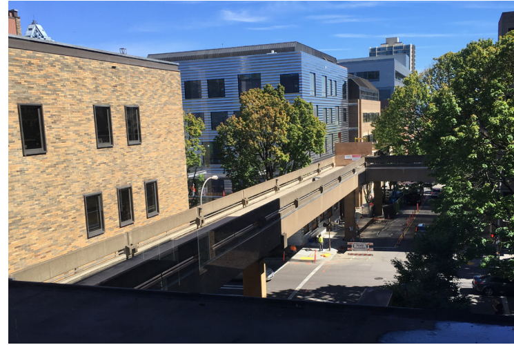
SW BROADWAY PEDESTRIAN BRIDGE FACING EAST
