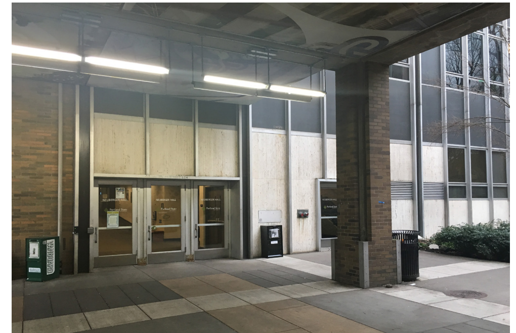
NORTH ENTRY DOORS
