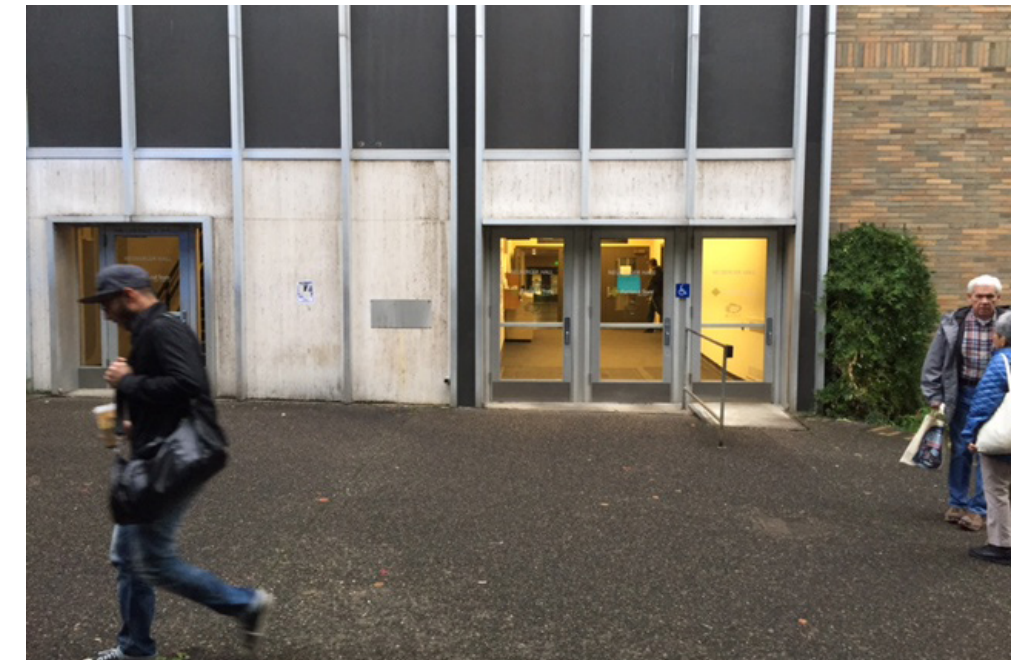
SOUTH ENTRY DOORS
