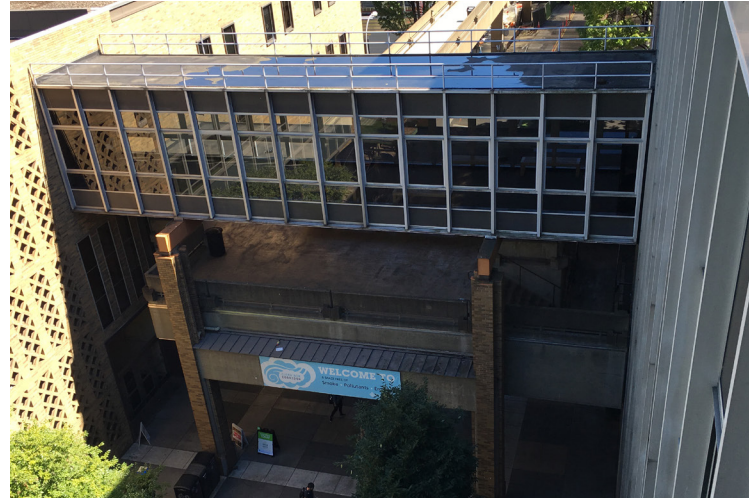
SW HARRISON ST PEDESTRIAN BRIDGES FACING EAST
