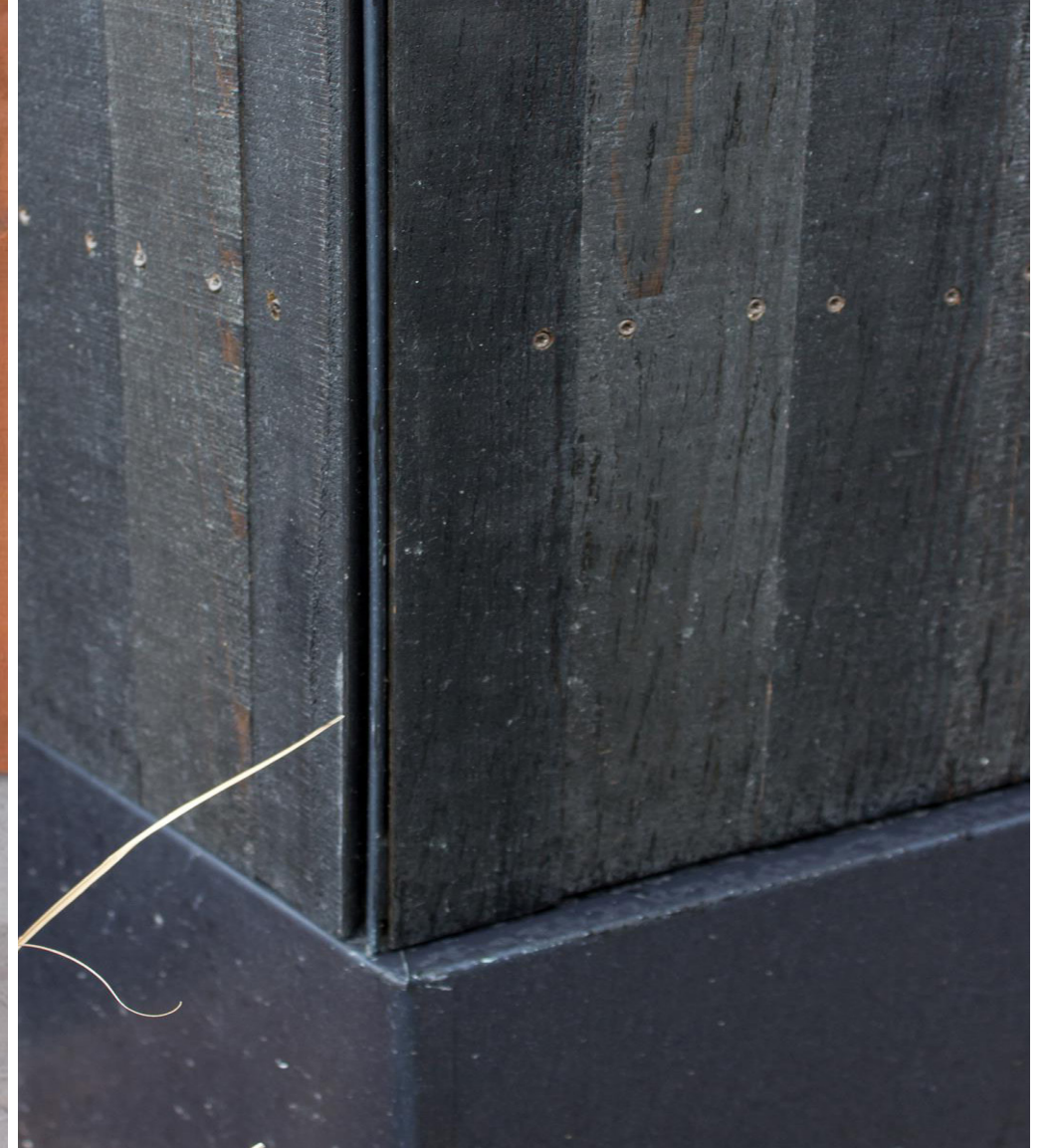
PROTECT CORNERS AND BOARD ENDS
