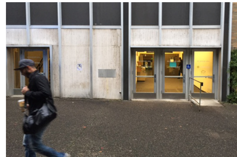
NEUBERGER HALL SOUTH BUILDING ENTRY
