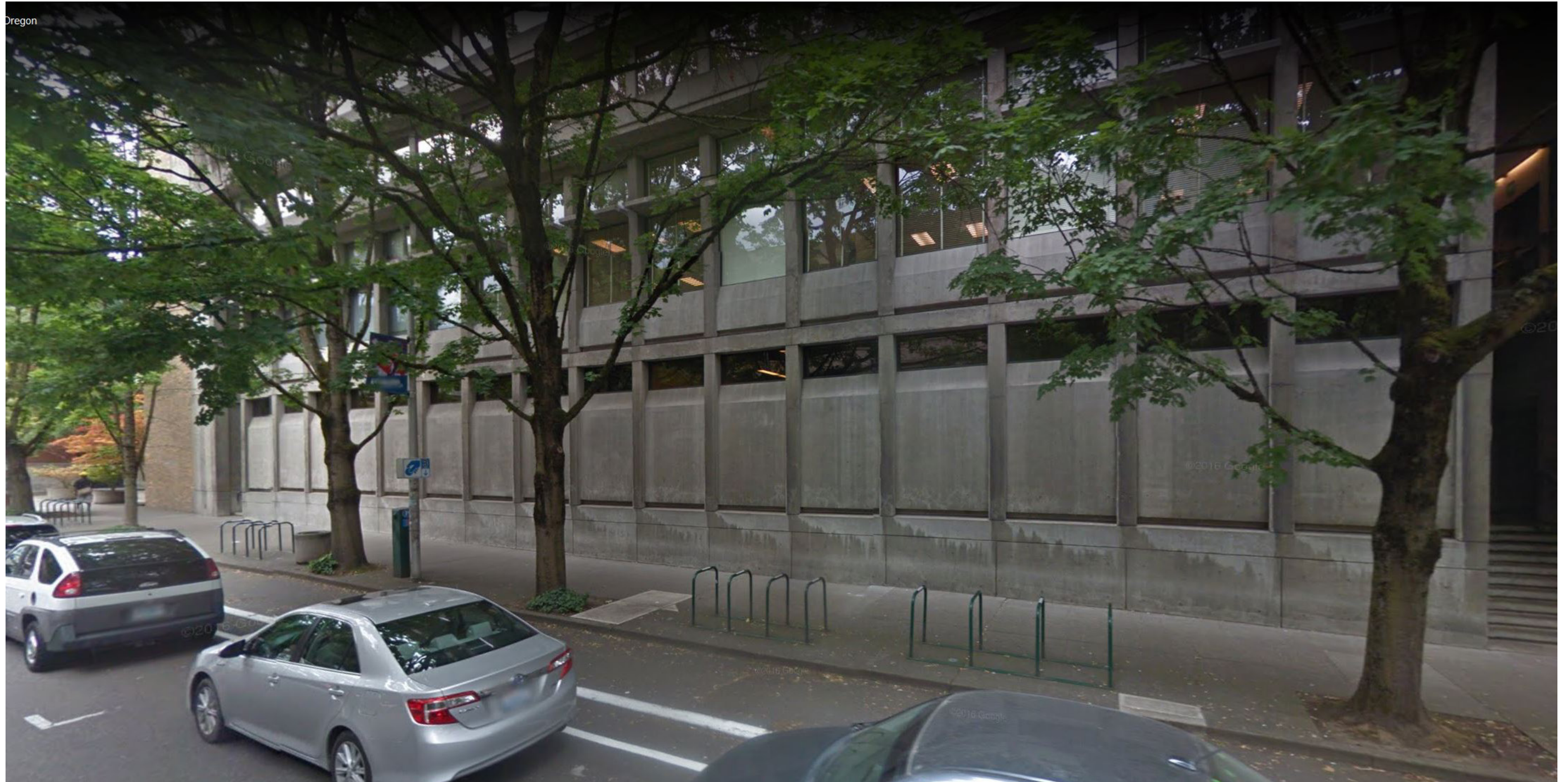
EXISTING EAST FACADE
